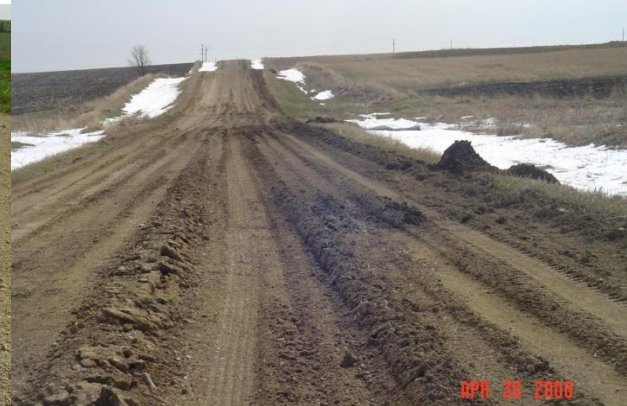
Figure 1. Unpaved roads and road condition. The images of top row show two roads in good condition. The roads shown in the images of the two middle rows demonstrate significant surface distresses, such as potholes, loss of crown, resulting water trapped on surface after rainfall which in turn further deteriorating roads in they are not properly repaired. The last row gives examples of roads with corrugation effects and severe rutting.
