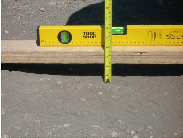
Measurement of ruts depth
