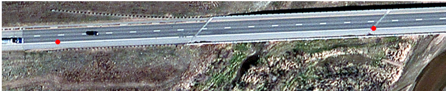
Mile 114.5-114.6, Fatigue 527 square meters
