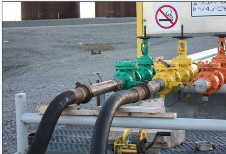
Figure10.4: Shore manifold
