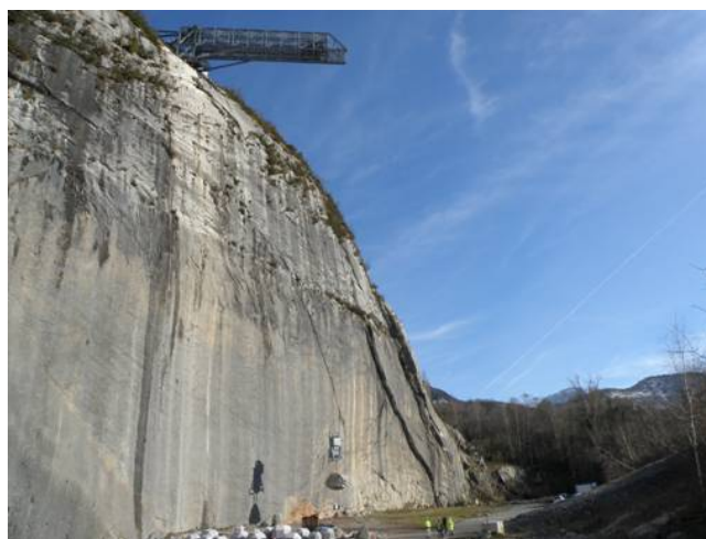
Figure 6. Global view of the LCPC rockfall test station.
