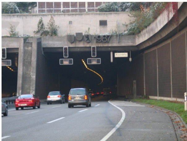
Figure 4-15: Rosenberg tunnel, portal east
