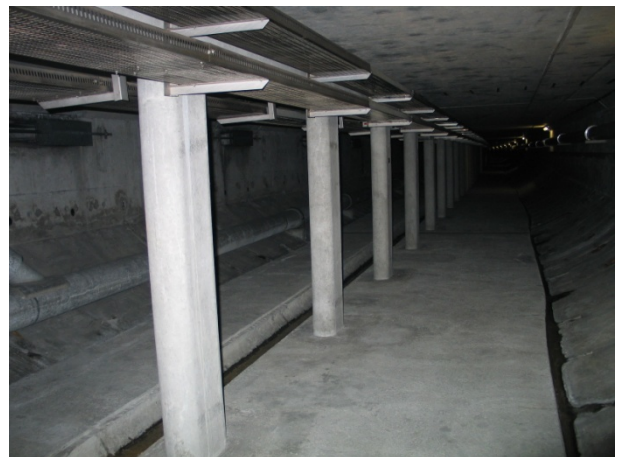
Figure 4-16: Rosenberg tunnel, beneath deck slab
