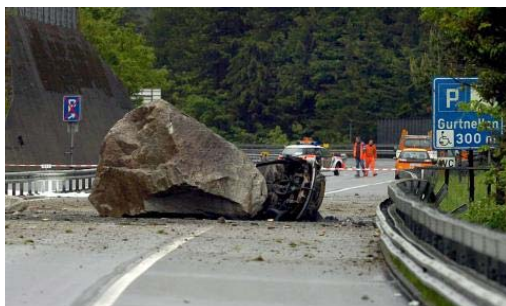
Figure 4-24: Rockfall on Gotthard motorway (A2), 2006
