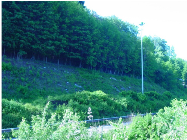
Figure 4-20: Schoren retaining wall
