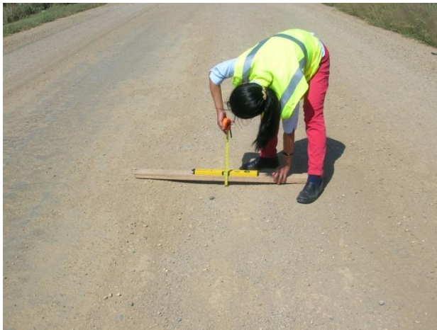
Measurement of pothole depth
