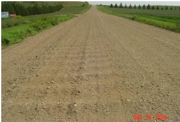
Figure 1. Unpaved roads and road condition. The images of top row show two roads in good condition. The roads shown in the images of the two middle rows demonstrate significant surface distresses, such as potholes, loss of crown, resulting water trapped on surface after rainfall which in turn further deteriorating roads in they are not properly repaired. The last row gives examples of roads with corrugation effects and severe rutting.
