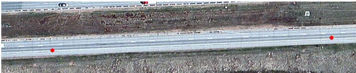
Figure 2: CDOT Highway Stretch #34A (Mile 114.8-114.9)
