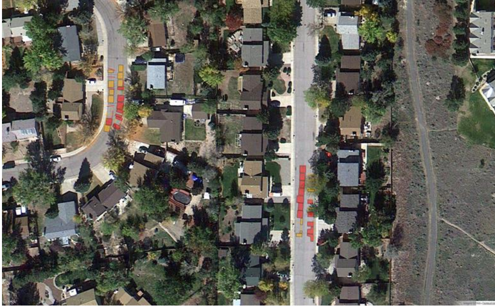
Figure 14: Google Maps Aerial Image with Road Damage Information
