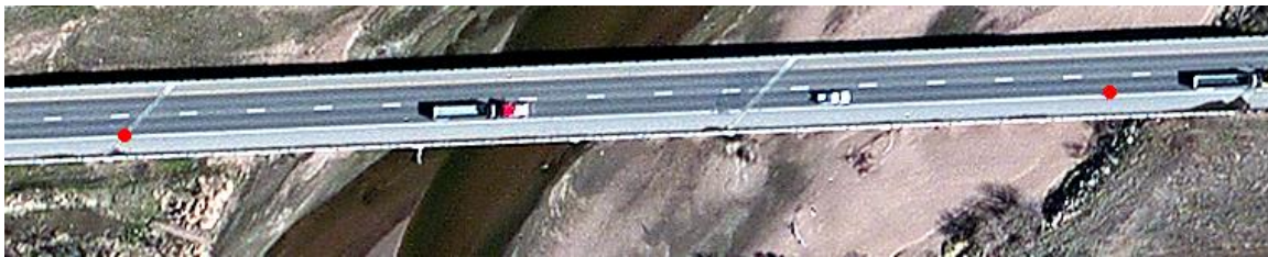
Figure 1: CDOT Highway Stretch #34A (Mile 114.6-114.7)
