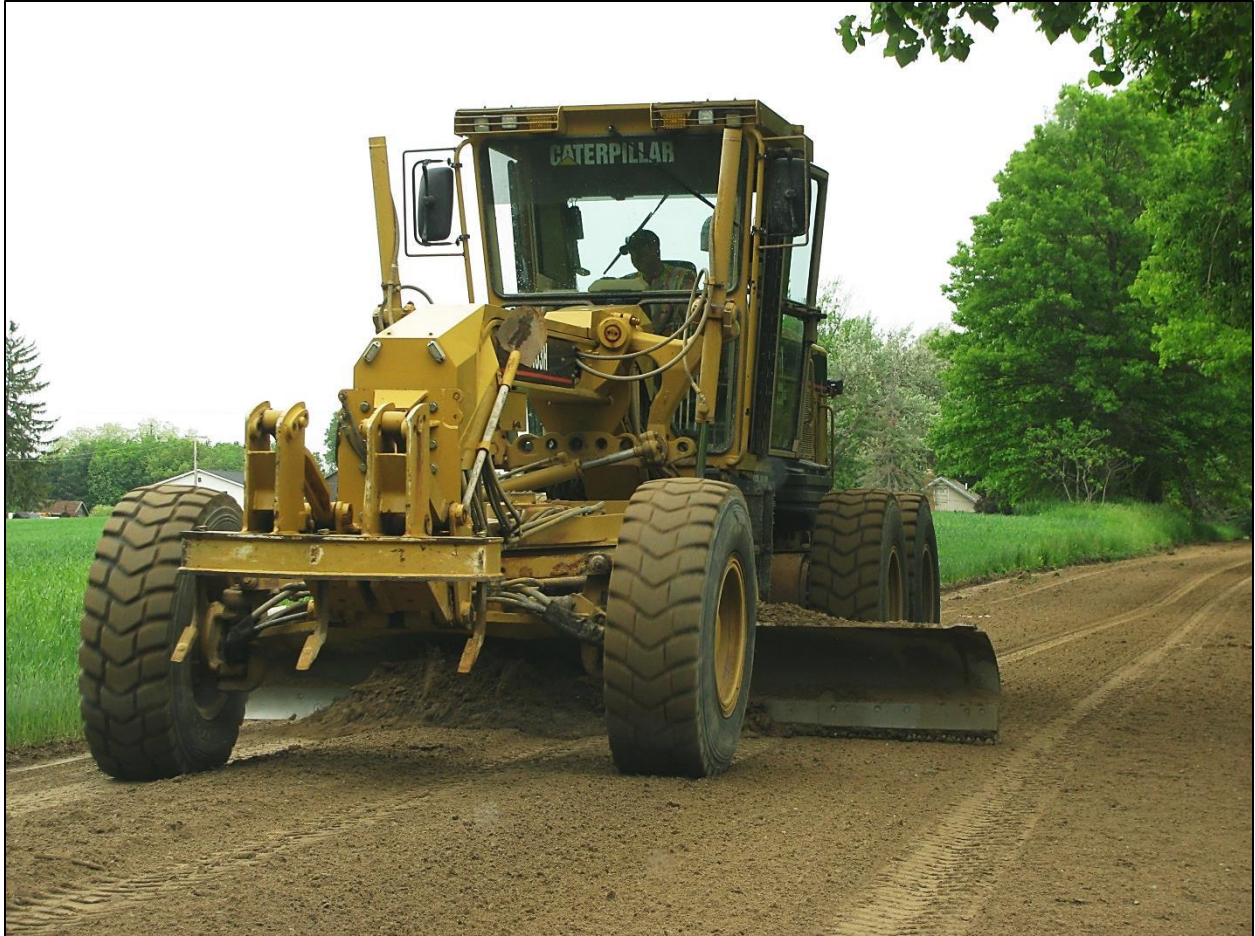
Figure 3: A road grader working on a rural road in Livingston County, MI, as seen by data collection team while looking for distressed unpaved roads.
