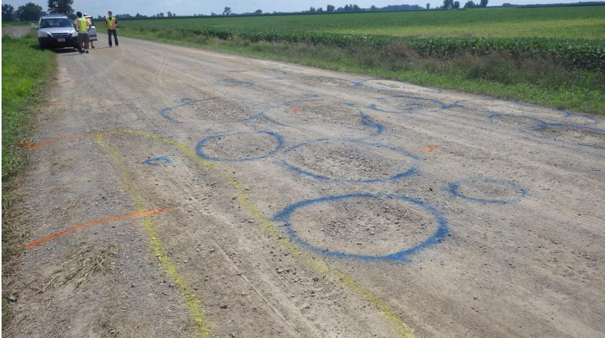
Figure 35: Piotter Hwy marked and measured during the 2013 data collection. Note the clustering of potholes at this particular location, which as a feature of the 2013 distress patterns (IMG0262.jpg)
