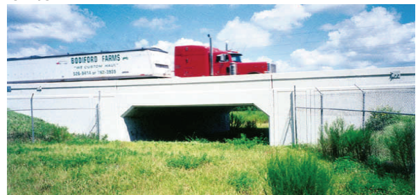
Animal crossing underpass with channelling fences. U.S. DOT
