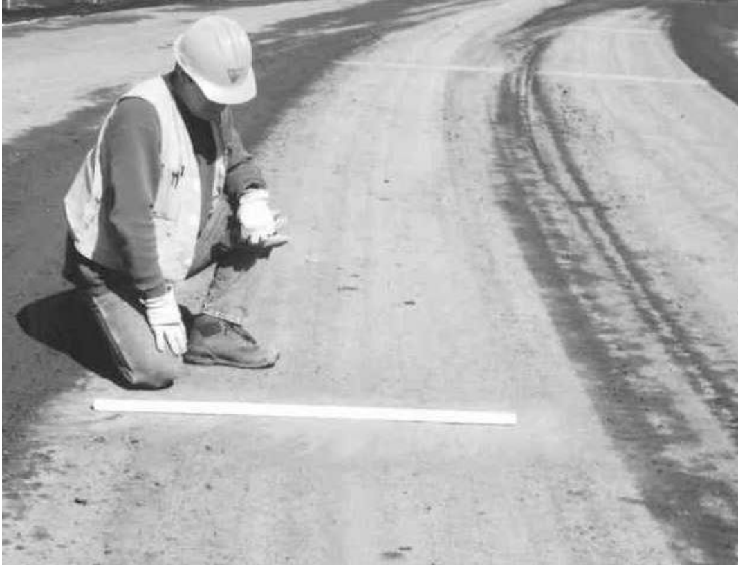
Figure 4.2 Rut Depth Measurement for the Pavement Condition Survey.
