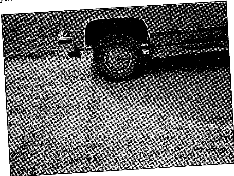
FIGURE 1b. Transverse Road View of Corrugations Longitudinal wave length corresponds approximately to footprint of 16-inch diameter tires.
