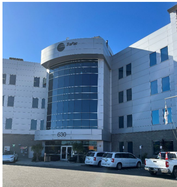
Figure 1. Trapac headquarters Long Beach, California (Photo courtesy of author)
