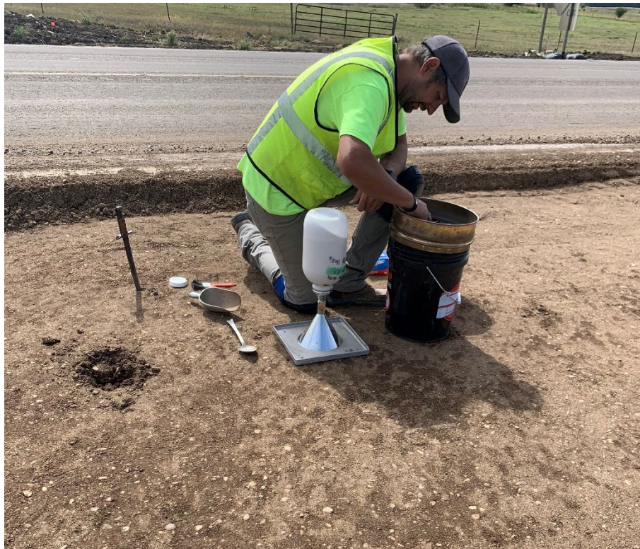
Figure 3.16 SCT Test being Conducted on an Aggregate Base (025D)
