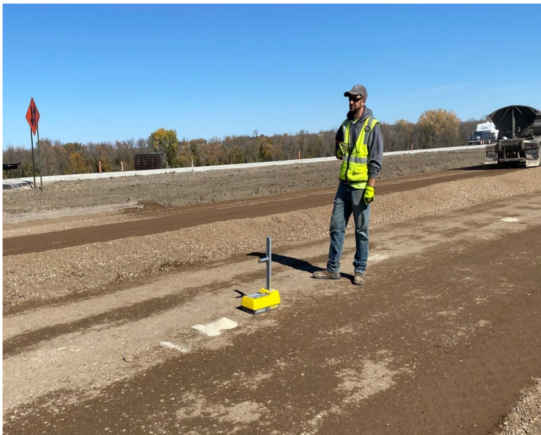
Figure 3.17 NDG Test being Conducted on an Aggregate Base (06DJ)
