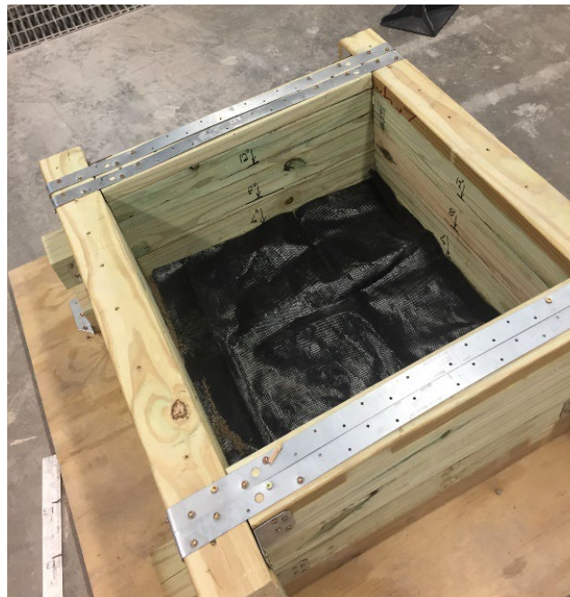
Figure 3.8 Compacted Sand Layer Covered by a Geotextile Layer in the Test Box
