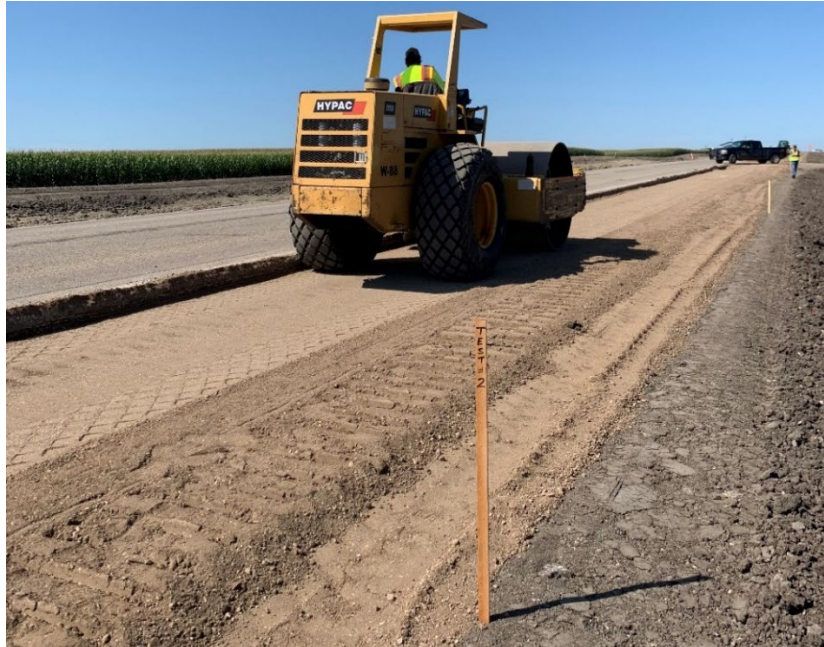
Figure 3.14 Compaction of a Base Layer (03RQ)
