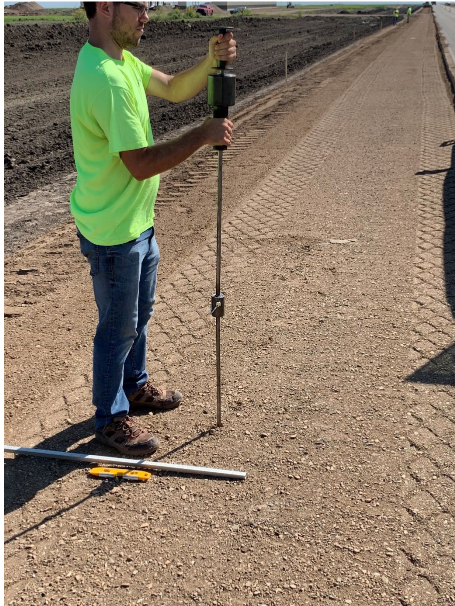
Figure 3.18 DCP Test being Conducted on an Aggregate Base (025D)
