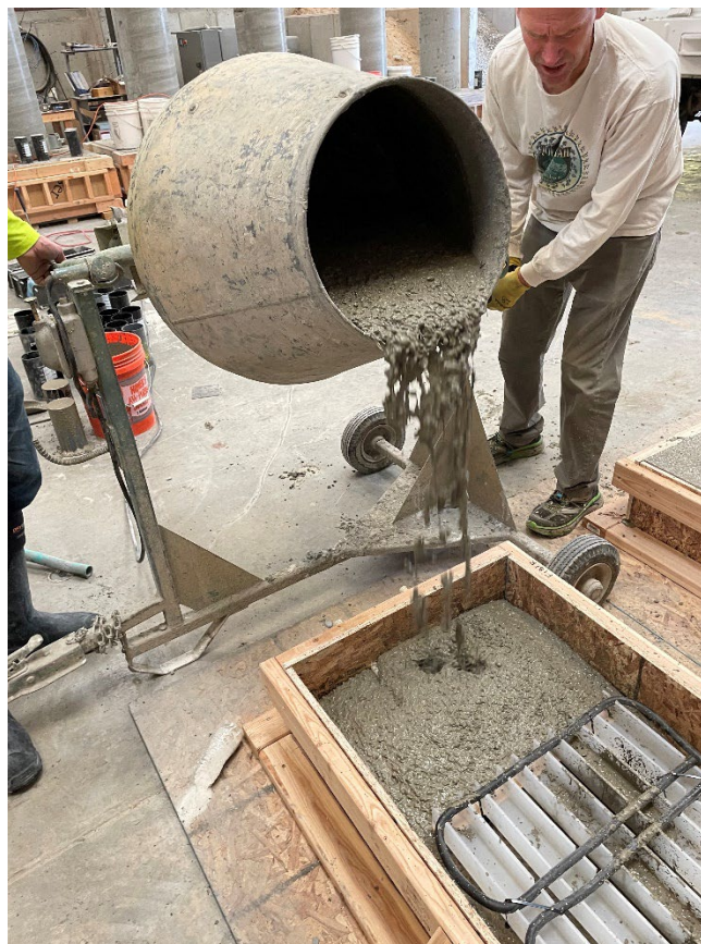
Figure 3.10 Pouring FRC Test Slab from Drum Mixer
