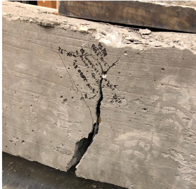
Figure 5.5 Steel Cracks at Failure
