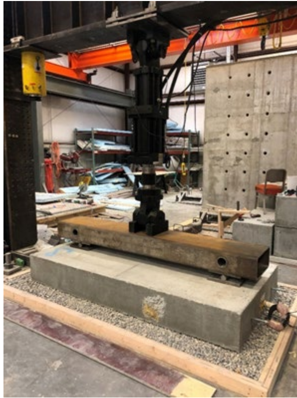
Figure 3.8 Finalized Testing Setup
