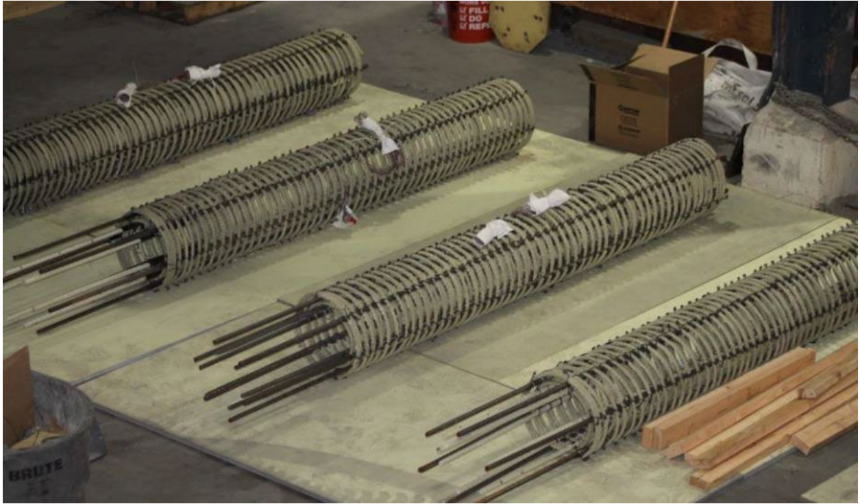
Figure 2.12 Column reinforcement cages
