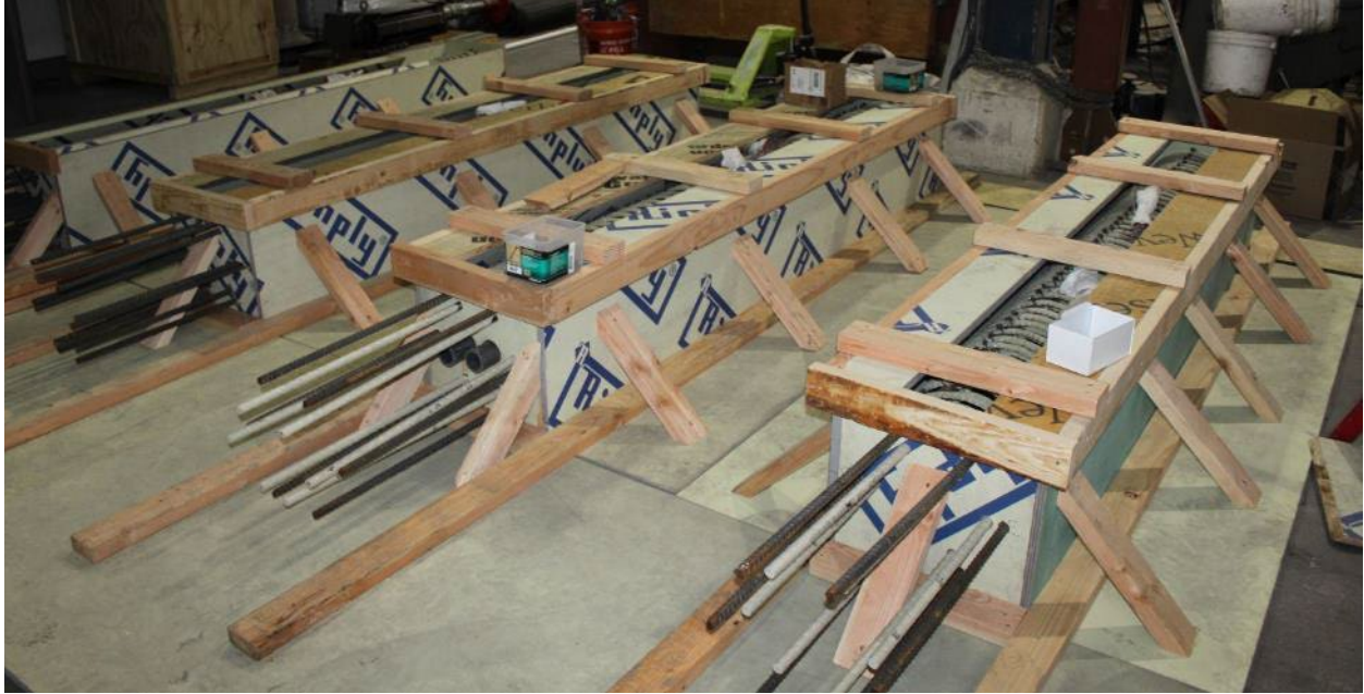
Figure 2.14 Column concrete casting formwork
