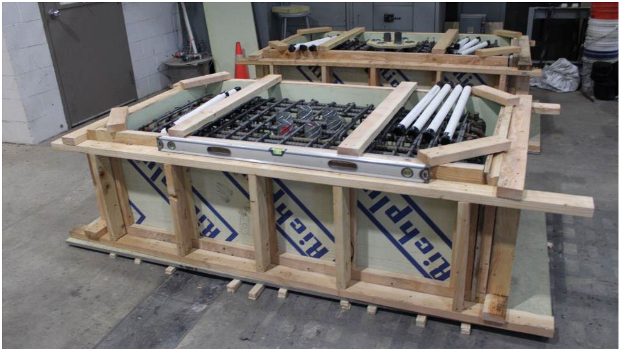
Figure 2.15 Footing concrete casting formwork
