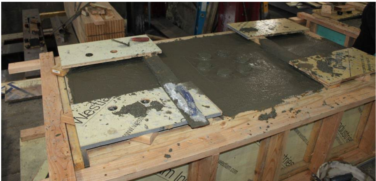
Figure 2.17 Footing concrete casting
