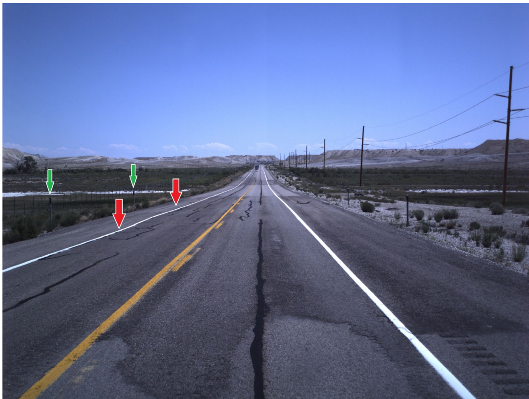
Figure 4.13 Photograph Looking Northbound (Positive Direction) of Patch Area with IRI Undulation in the Negative Direction of Travel Indicated by Red Arrows. Culvert Markers are Indicated by Green Arrows. (Courtesy of UDOT/Mandli Communications)
