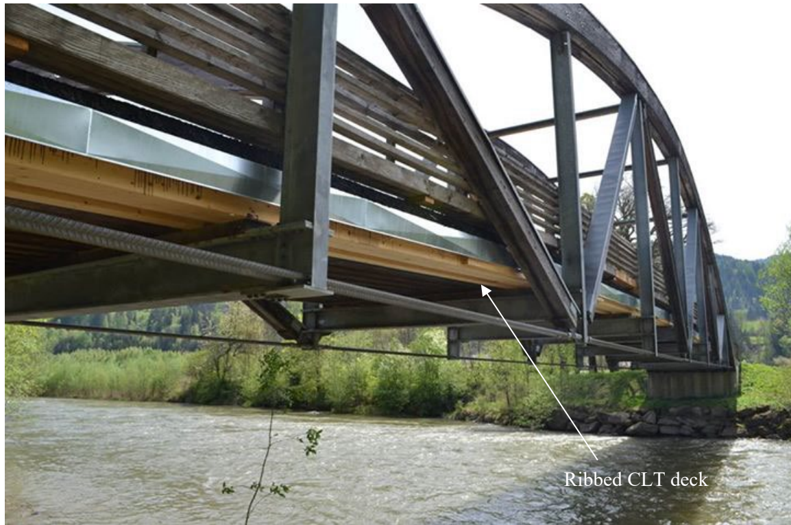
Figure 2.4 Arch bridge with CLT deck over River Mur, Austria (Behrens and Benner 2015)
