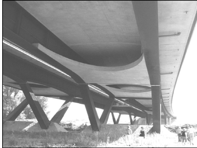
Figure 2.11 Odra River bridge, Czech Republic (PAŇTAK 2012)
