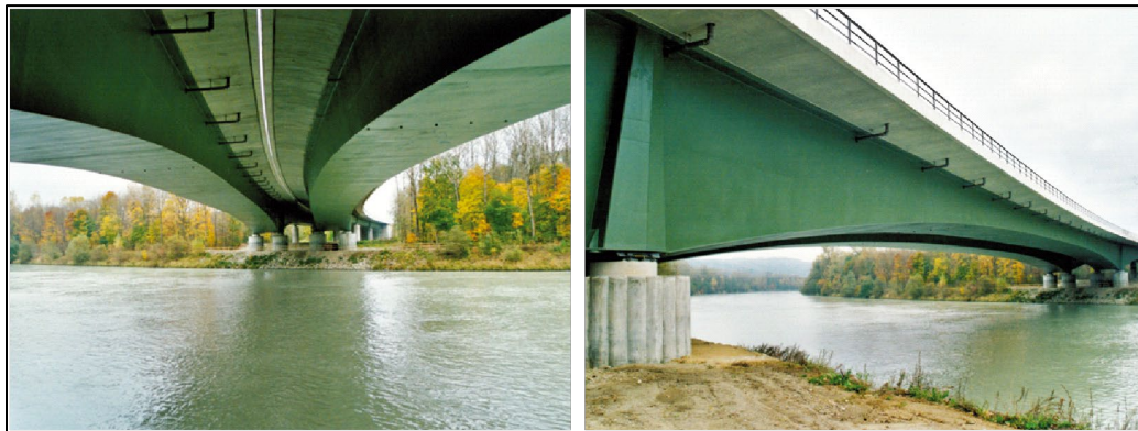
Figure 2.14 Inn River in Neuötting bridge, Germany (PAÑTAK 2012)
