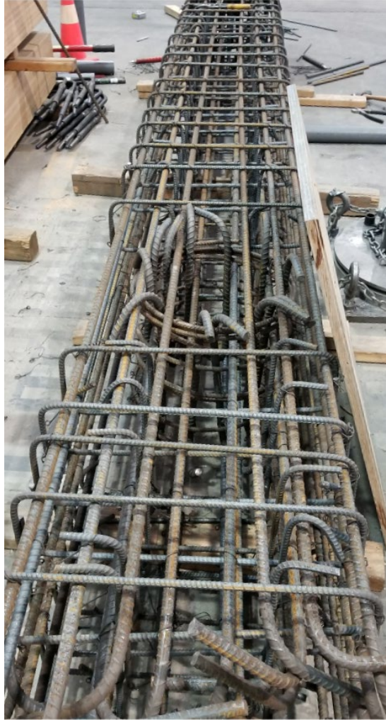
Figure 3.3 Reinforcement cage of cap beam
