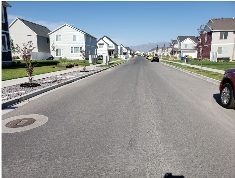
Figure 3.5 Section UT-07 showing no visible distresses
