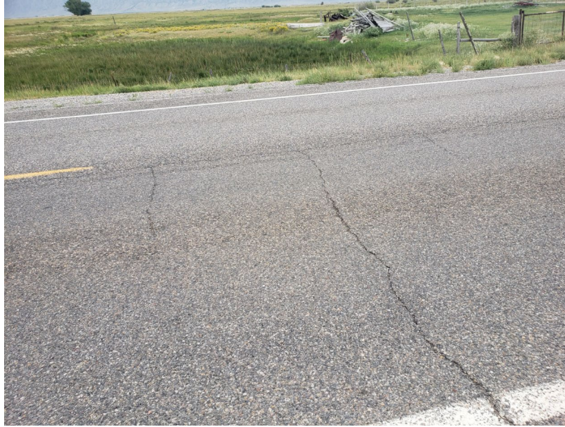
Figure 3.2 Section UT-03 showing thermal and reflective cracking
