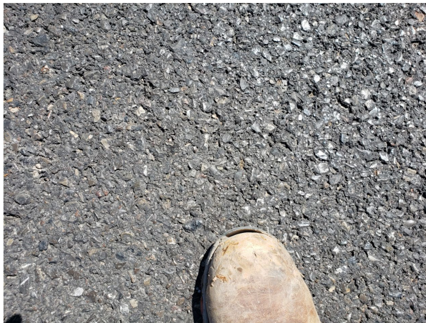
Figure 3.1 Section UT-02 showing fatigue cracking and raveling
