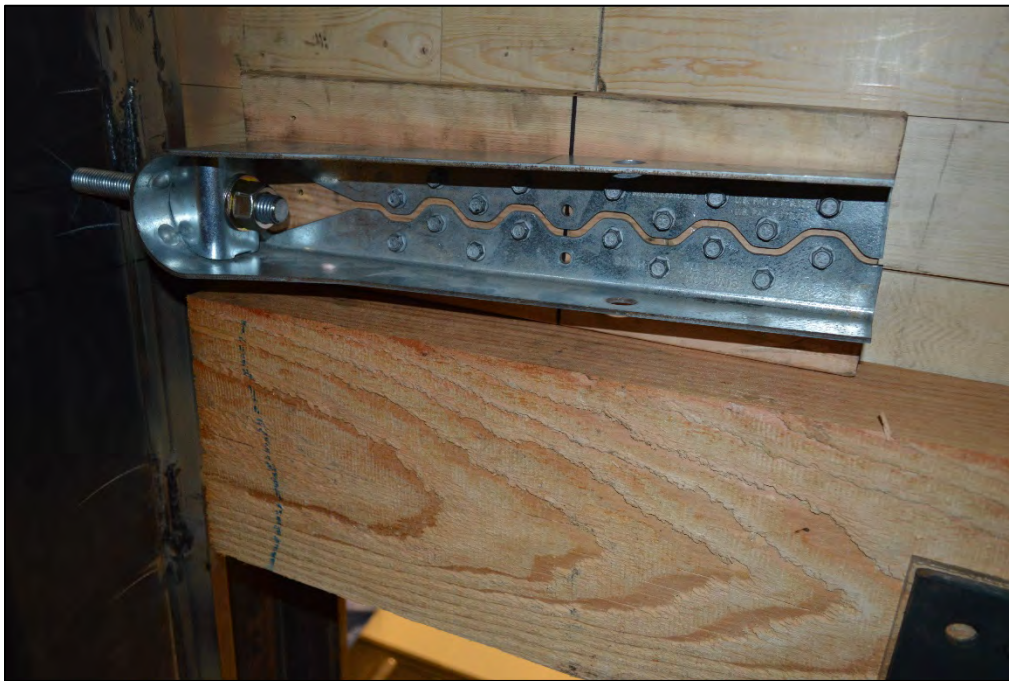
Figure A.19 HDU Hold-down
