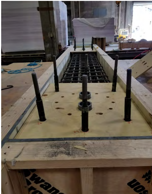
Figure 3.7 Construction details of the cap-beam
