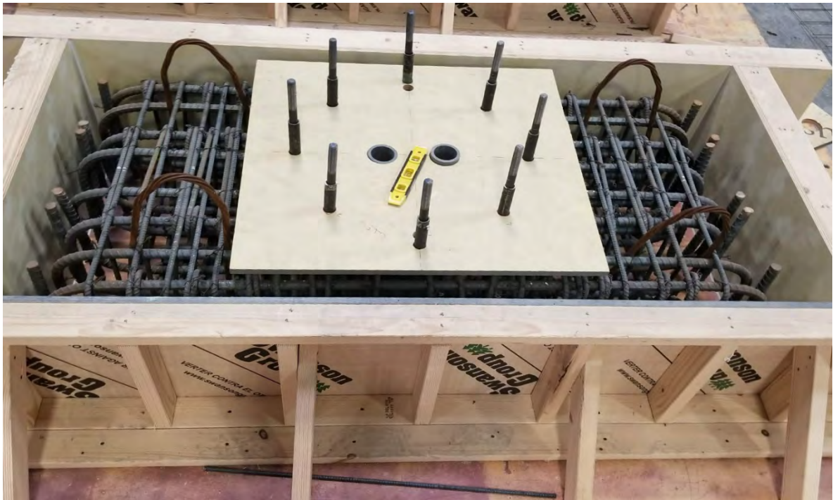
Figure 3.15 Construction details of the footing
