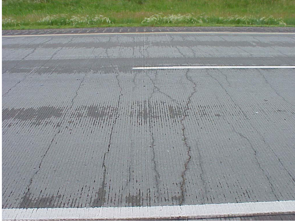
Figure 3.1 Network and Y-cracking (Johnston 2009)
