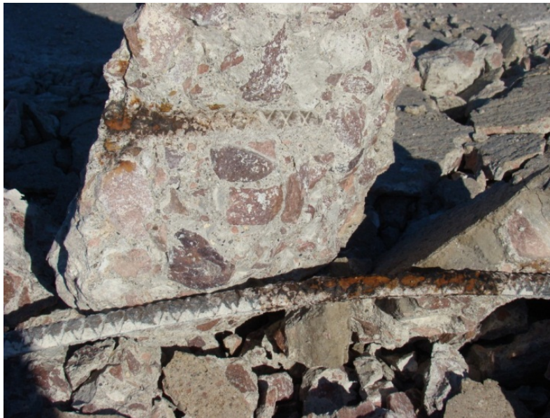
Figure 5.23 Localized corrosion found in the concrete rubble that was eventually removed
