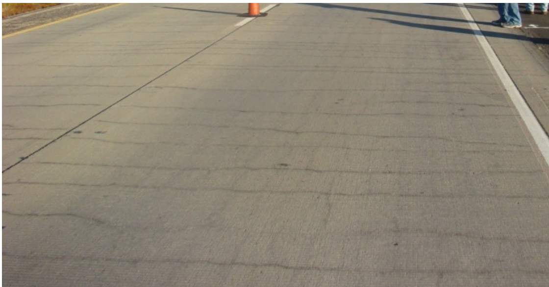
Figure 5.1 Cracking on Interstate 29 at MRM 87
