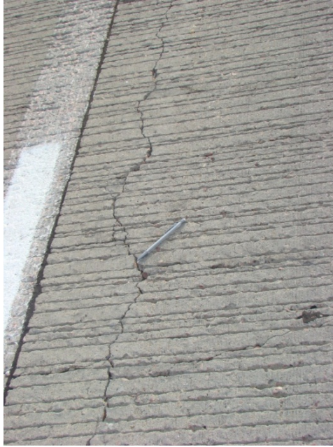
Figure 5.27 Longitudinal cracking on I-90
