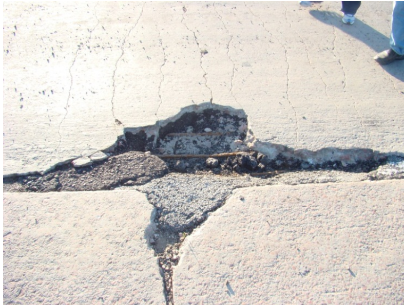
Figure 5.22 Patched pavement with exposed reinforcing steel
