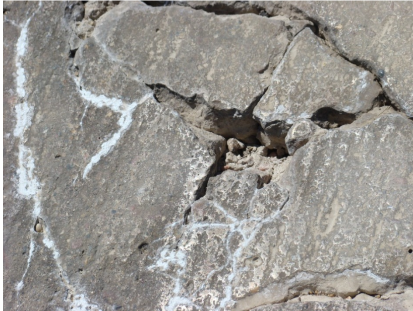
Figure 5.24 Spalled area with no signs of corrosion
