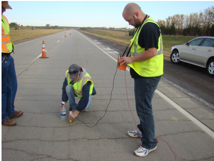
Figure 4.8 Collecting half-cell measurements
