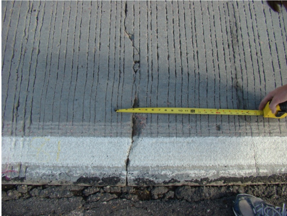
Figure 5.37 Wide crack exhibiting spalling at MRM 222
