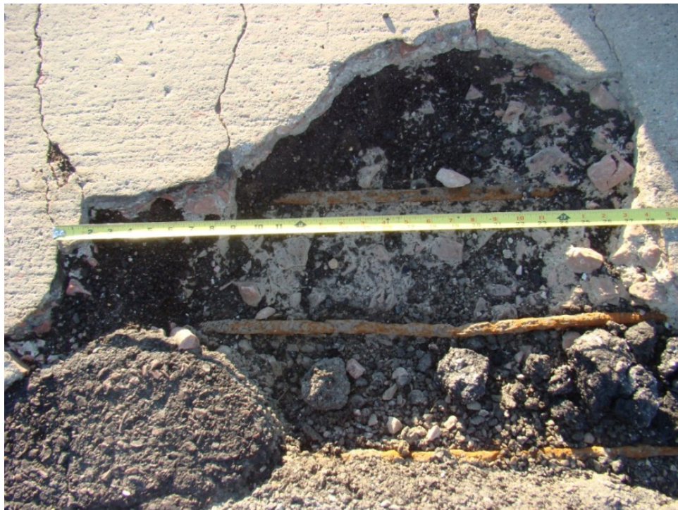
Figure 3.3 Corroded reinforcement exposed during CRCP removal
