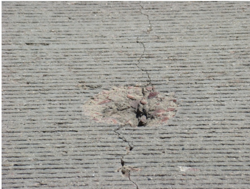
Figure 5.33 Spalling observed in passing lane at MRM 44
