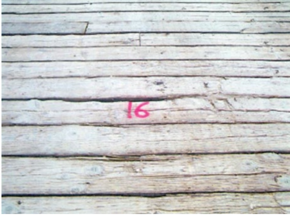
(g) Crack in 16 th plank from north prior to replacement
