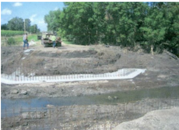
(q) Abutment wall reinforcement
