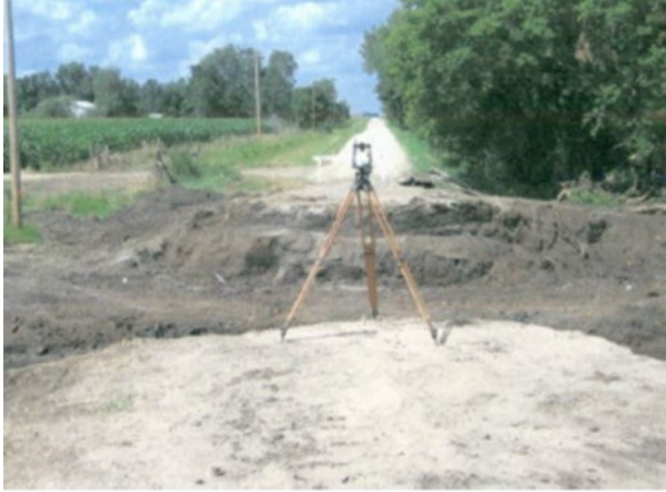
(m) Preparing site for abutment construction
