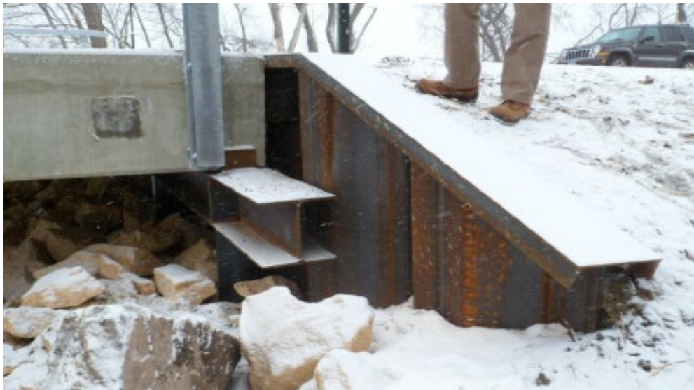
Figure 4.10 Sheet pile abutment (MnDOT, 2012)
