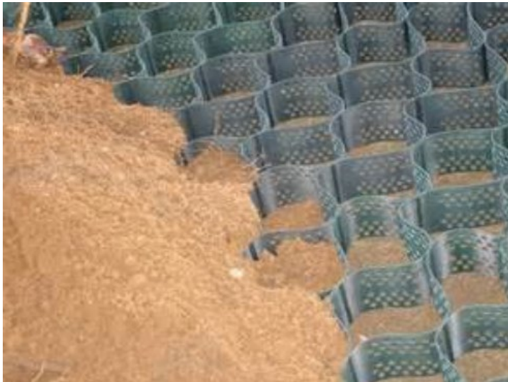
Figure 4.13 Cellular confinement system (CCS) (Cell-Tek, 2010)
