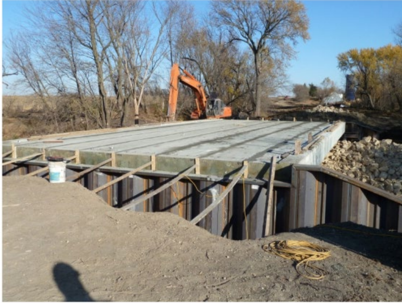
Sheet Pile Abutment
