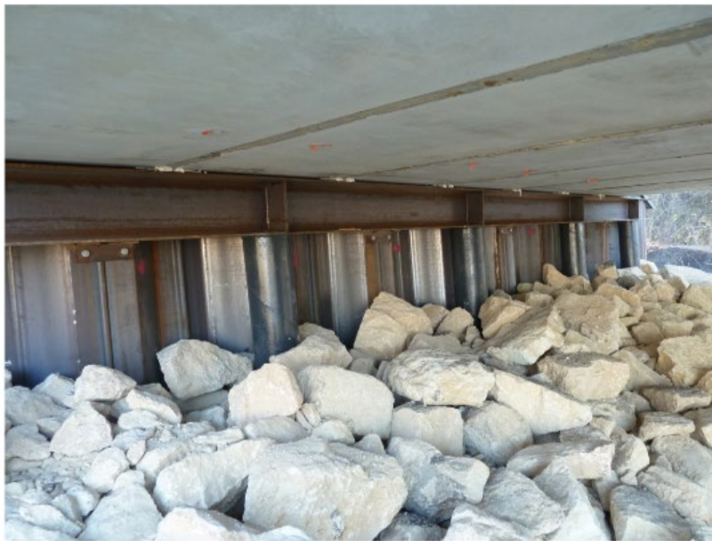
Sheet Pile Abutment
