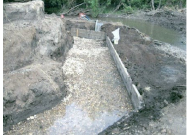
(n) Gravel placement prior to installation of reinforcing
