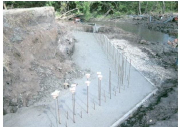
(p) Concrete placement with abutment reinforcement
