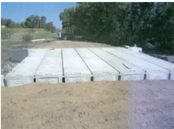
(w) Placement of adjacent box slabs
