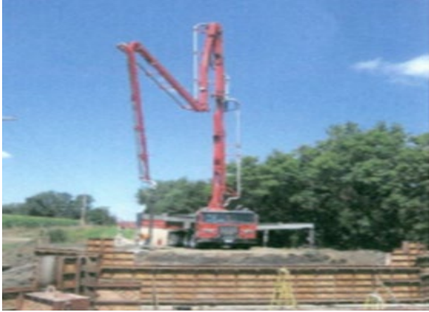
(s) Placement of abutment wall concrete
