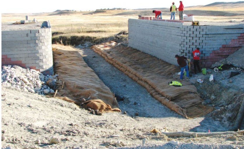
Geosynthetic Reinforced Soil (GRS) Abutment
