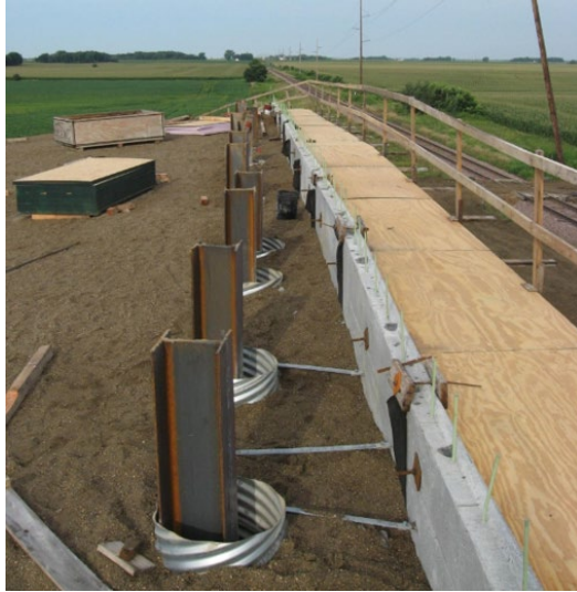
Abutment Piles in a Straight Line
