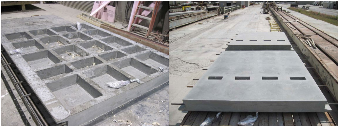
UHPC Waffle Bridge Deck Panels (Heimann, 2013)
