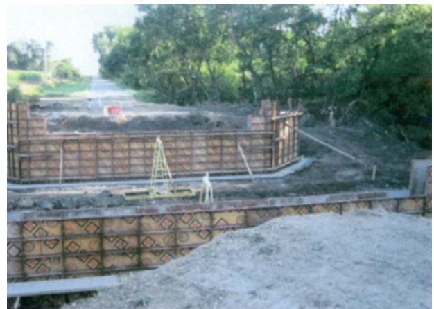
(r) Abutment wall formwork
