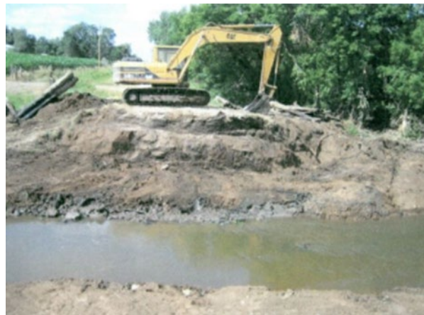
(k) Preparing site for abutment construction
