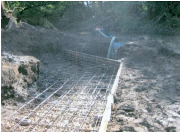
(o) Abutment footing reinforcement
