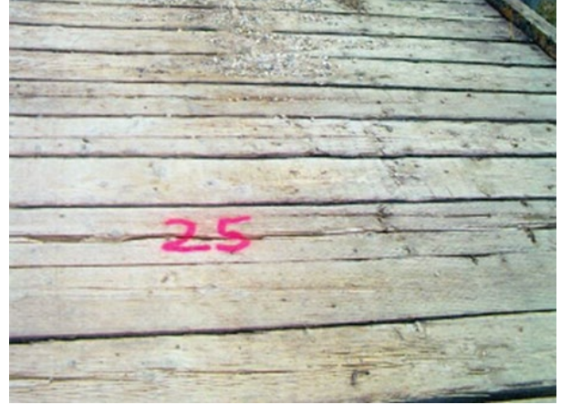
(h) Crack in 25 th plank from north prior to replacement
