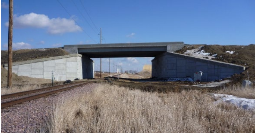
Figure 4.9 Geosynthetic reinforced soil (GRS) abutment (MnDOT, 2012)
