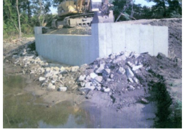
(t) Abutment backfill and riprap placement
