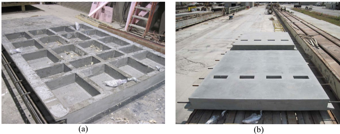
Figure 4.6 UHPC waffle bridge deck panels. (a) bottom side of panel (Heimann 2013) (b) top side of panel (Heimann, 2013)
