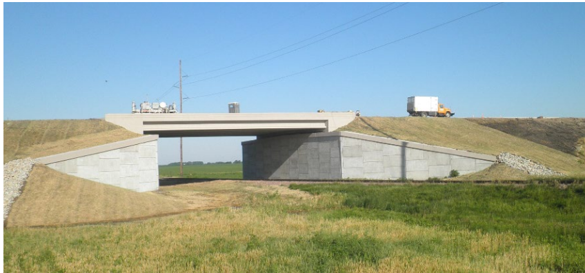
Mechanically Stabilized Earth (MSE) Wall
