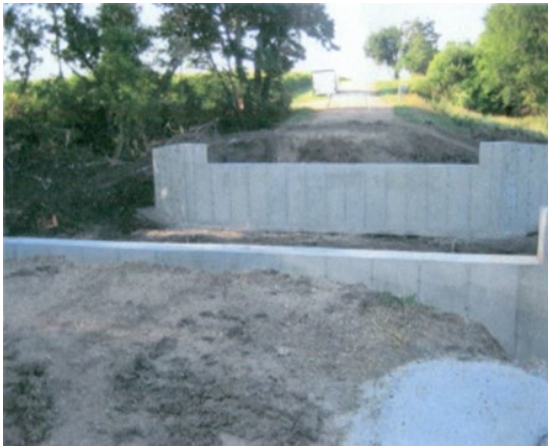
(u) Completed abutments
