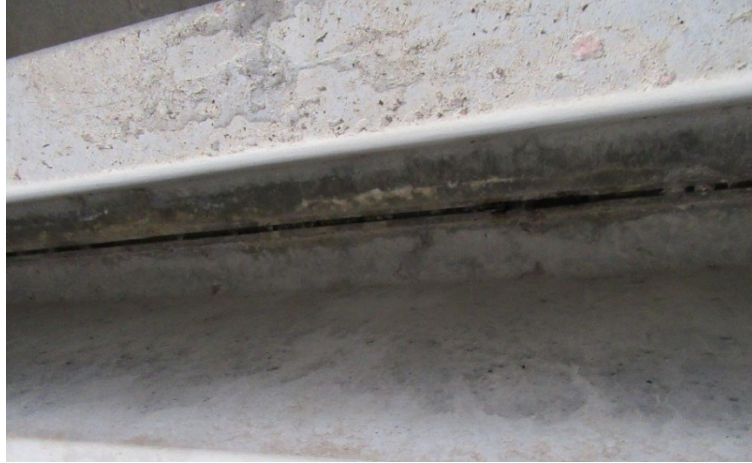
Figure 3.3 Efflorescence and erosion between G7 and G6 on Bridge A (Credit: Brian Kidd)
