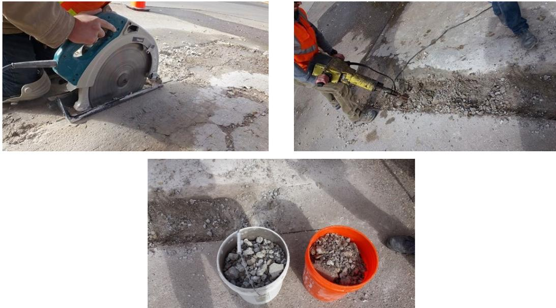
Figure 3.1 Process of collecting RCA aggregates
