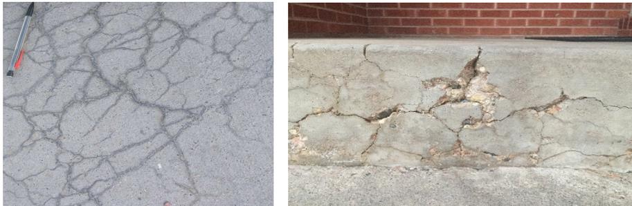
**Figure 2.3** ASR damage in Wyoming a) map cracking at Federal Street in Riverton and b) pop-outs combined with map cracking in Cheyenne
