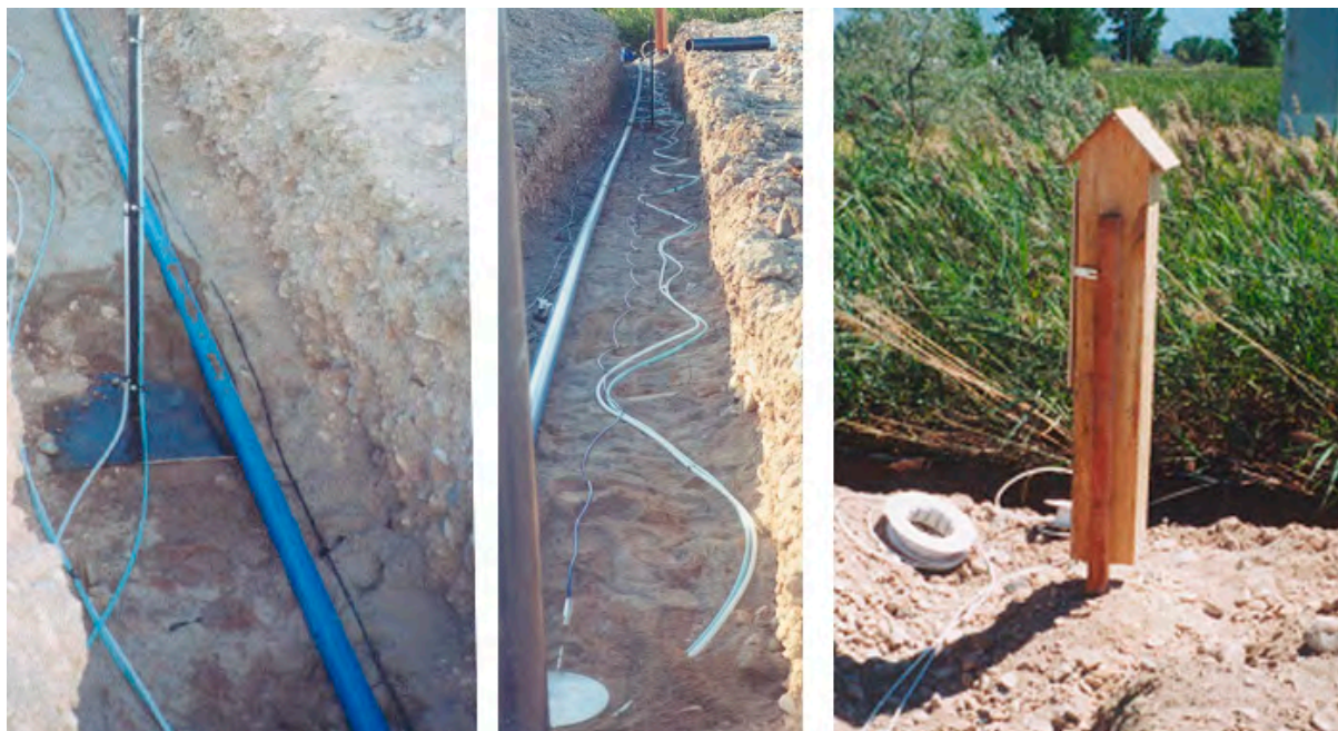
Figure F10. Settlement manometer standpoint (left). Plastic tubing (center). Housing box with measuring staff inside (right). Note inclinometer casing and pressure cell have also been installed at this site.
