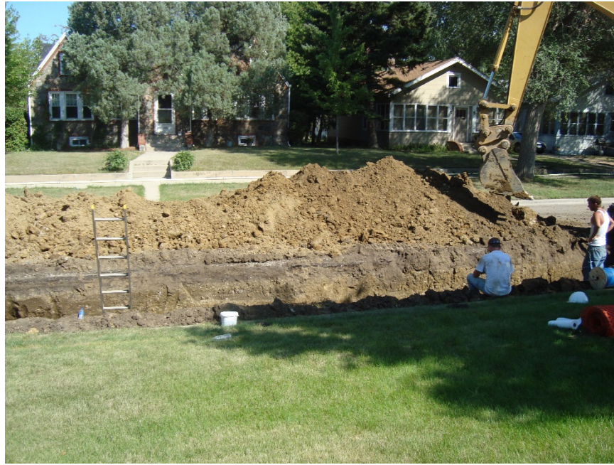
Figure 3.1 Aberdeen construction site
