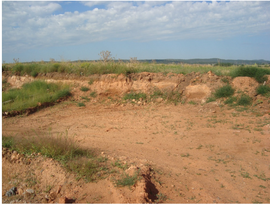
Figure 3.14 Rapid City construction site
