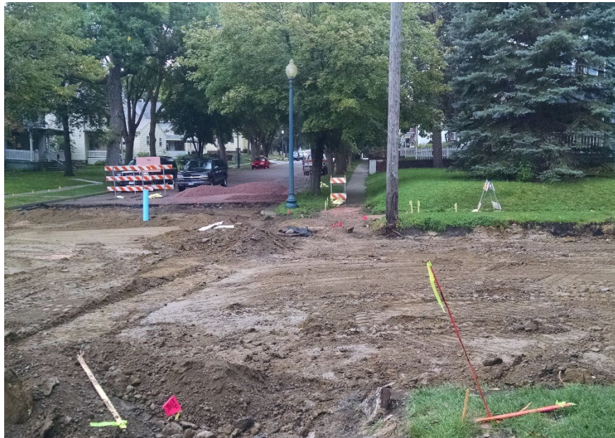
Figure 3.2 Sioux Falls construction site
