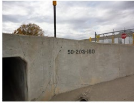
Cracking in the Wing Walls
