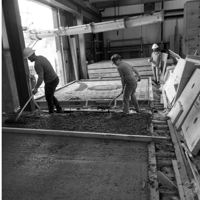
**Figure 4.3.5** Pouring the GFRP punching shear decks
