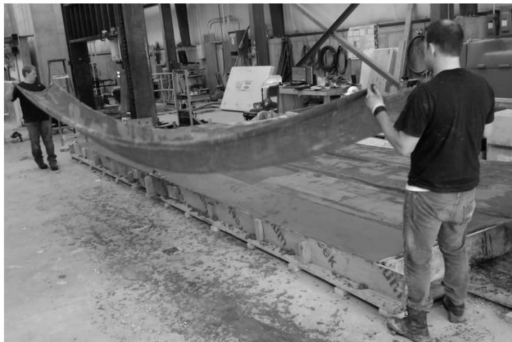
**Figure 3.3.7** Laying moist burlap on the panels
