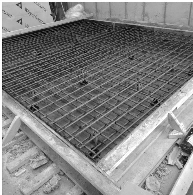
**Figure 4.3.2** Steel punching shear deck prior to pouring
