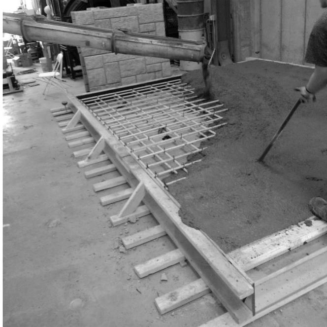
**Figure 4.3.7** HRC decks being poured with internal vibration
