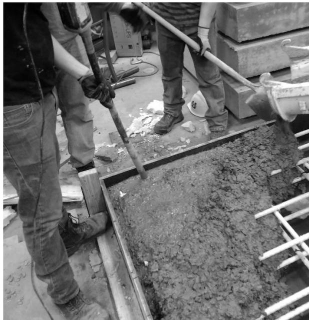
**Figure 3.3.5** Internal vibration of deck panels
