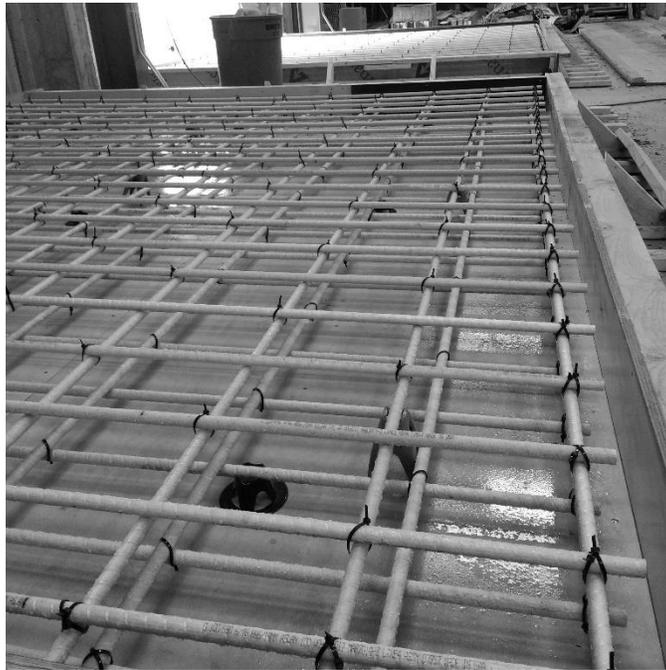
**Figure 4.3.6** HRC punching shear decks before casting
