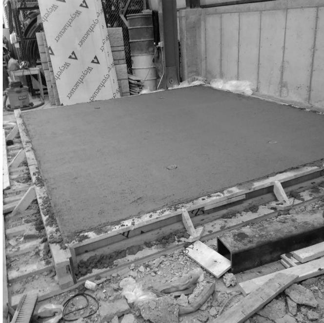
**Figure 4.3.8** Finished GFRP punching shear deck
