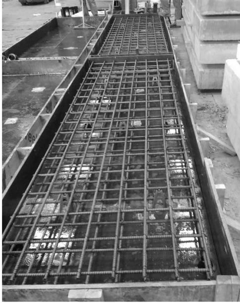
**Figure 3.3.6** Steel-reinforced decks prior to pouring
