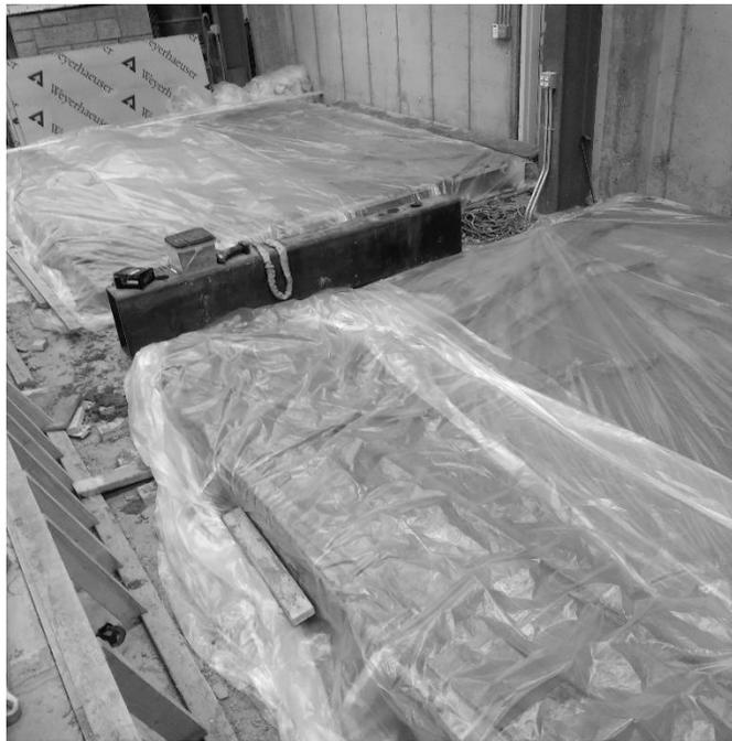
**Figure 4.3.9** Curing the punching shear decks
