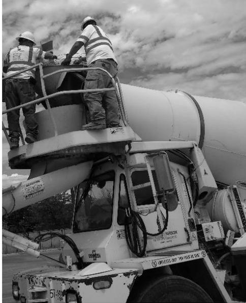
**Figure 4.3.1** Adding the fibers at the batch plant
