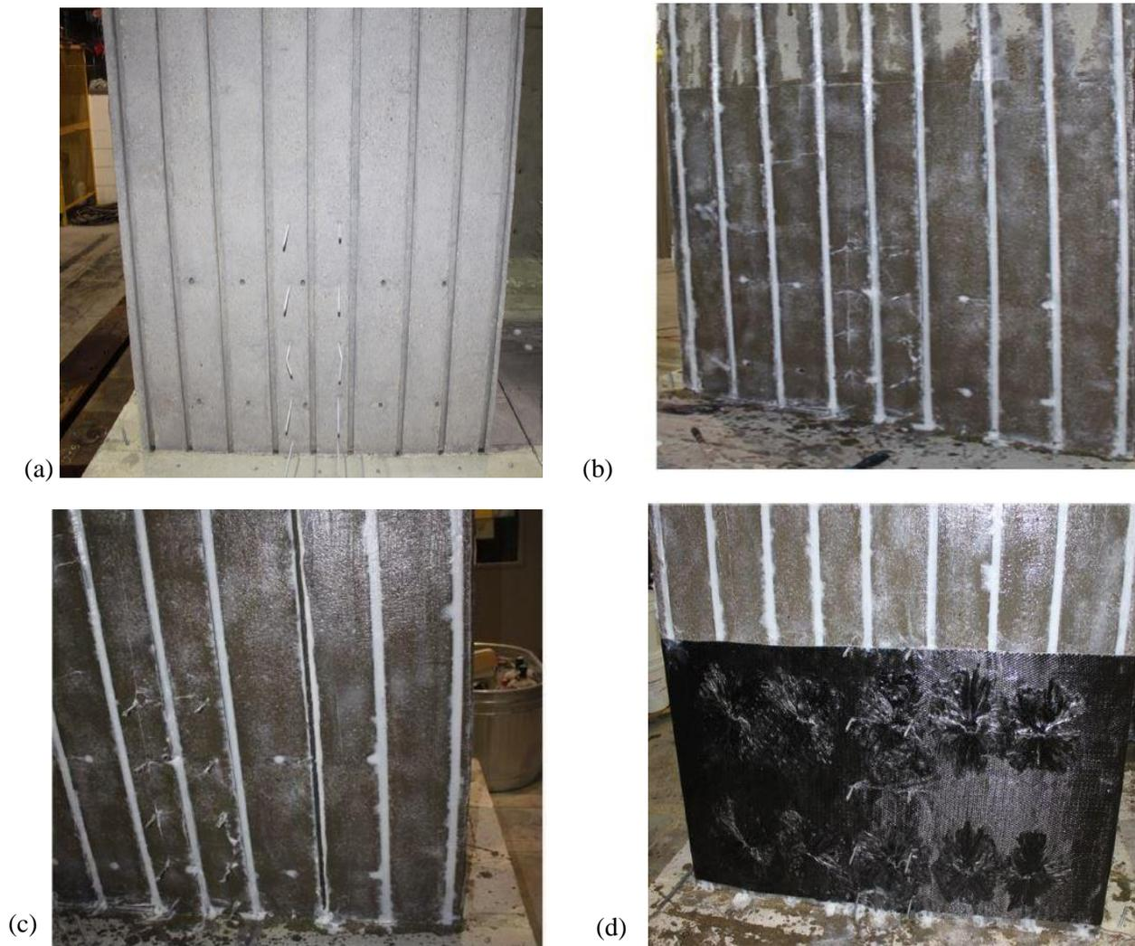
**Figure 6.2** Retrofit process for specimen R2: (a) sandblasted surface, (b) application of premixed epoxy, (c) installation of CFRP NSM rods, (d) CFRP wrap and installation of CFRP horizontal anchors
