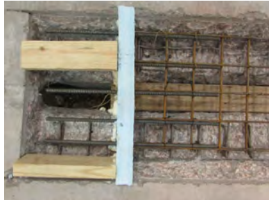
c. Block-out Formwork
