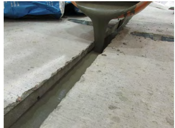
b. Grouting Girder-to-Girder Keyway
