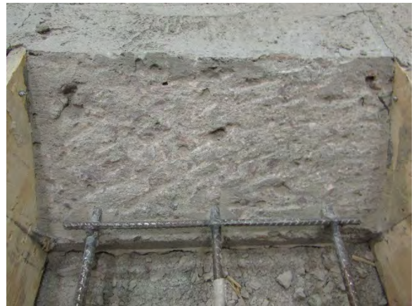
d. Roughened Joint Surface
