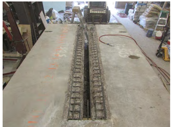
b. Continuous Joint Preparation – Segment II
