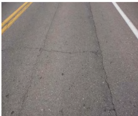
a. Reflective Cracking of Asphalt Overlay
