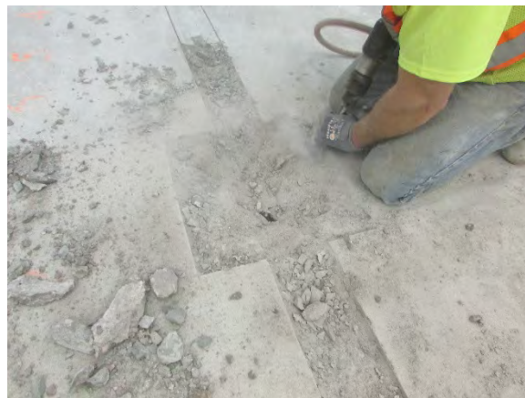
e. Pocket Demolishing
