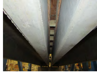
b. Underneath View, Continuous Joint Segment I Formwork
