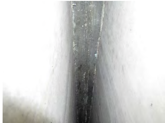
b. UHPC Pocket Joint - Underneath Bridge
