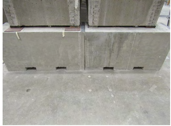
b. Placement on Abutment
