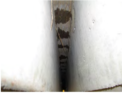
a. Leak in LMC before Testing
