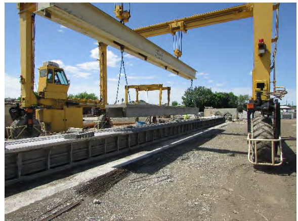
d. Removal from Formwork
