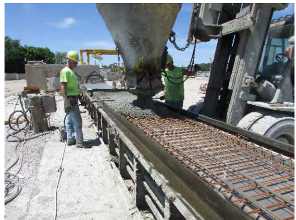
b. Concrete Casting
