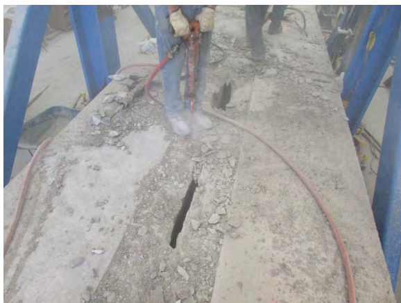
c. Continuous Joint Demolishing – Segment I
