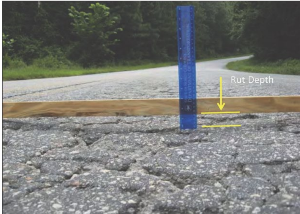
Figure 2.6 Pavement Rutting (Serigos et al., 2012)
