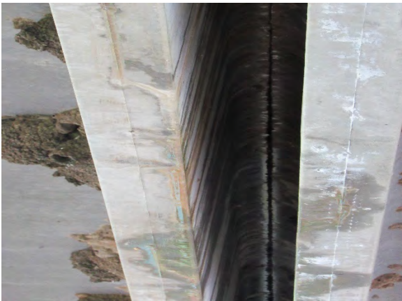
(e) Efflorescence
