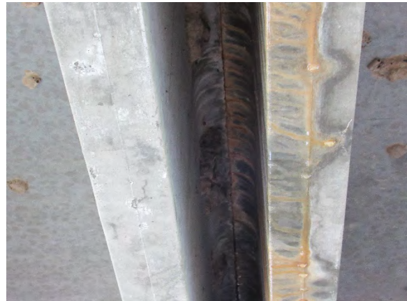
(f) Sign of corrosion
