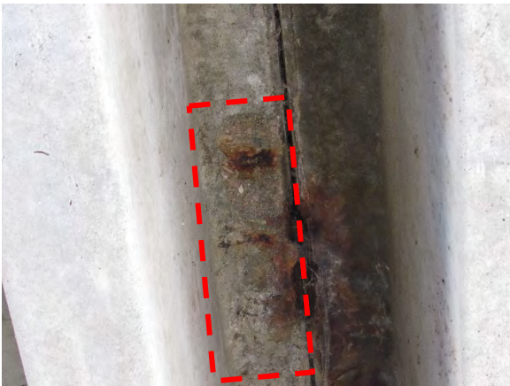
(e) Deterioration in Joint
