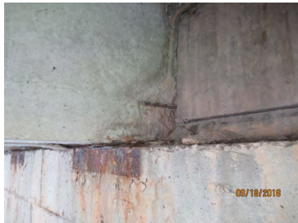
(e) Spall with Prestressing Strand Exposed – South End of East Stem of Deck Unit 3
