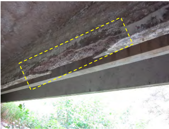
(a) Stem Cover Deterioration
