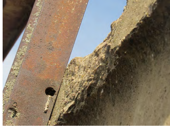
(b) Deterioration at side of bridge
