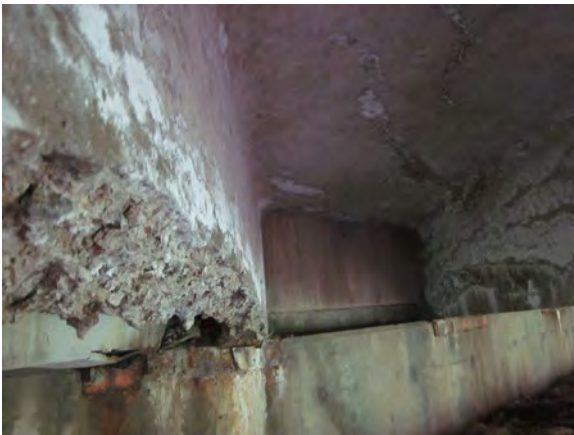
(a) Underneath View of Girder
