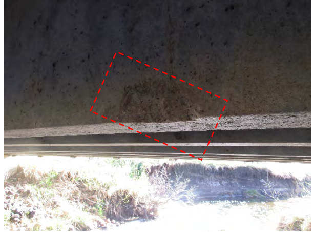
(b) Spalling at bottom of Stem, G4
