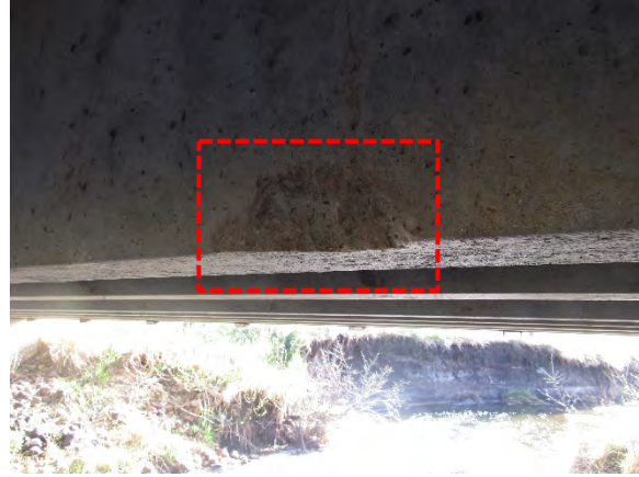
(b) Spalling at stem of bridge
