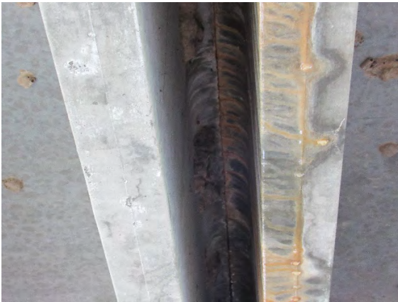
(c) Girder-to-Girder Damage
