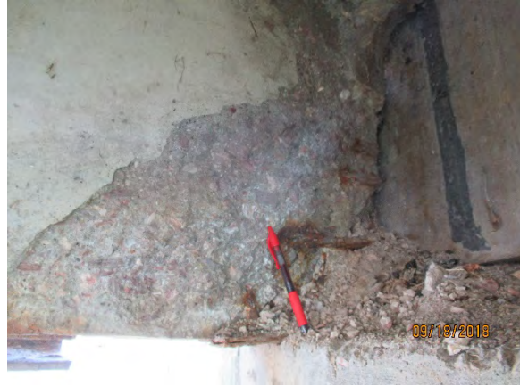
(g) Spall with Prestressing Strand Exposed – South End of East Stem of Deck Unit 7
