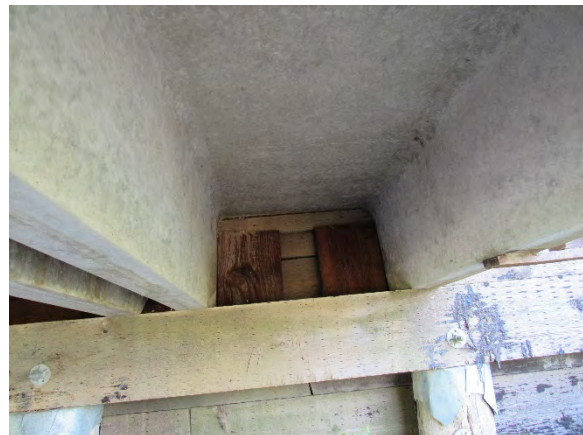
(f) Wooden diaphragm at end of girder
