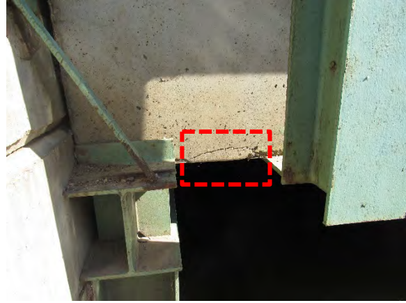
(b) Cracking at bottom of exterior girder
