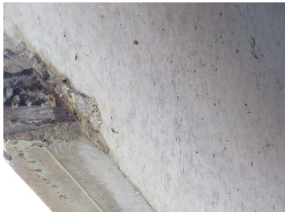
(f) Deterioration at bottom of stem
