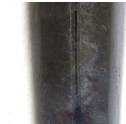
(c) Efflorescence in joint
