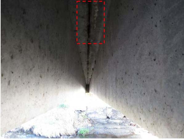
(a) Efflorescence in Joint
