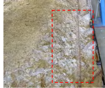
(f) Flange Cover Deterioration (CS-4)
