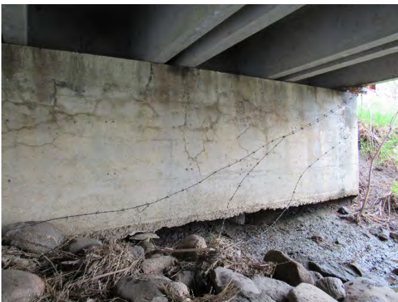
(e) Scouring from bottom of abutment
