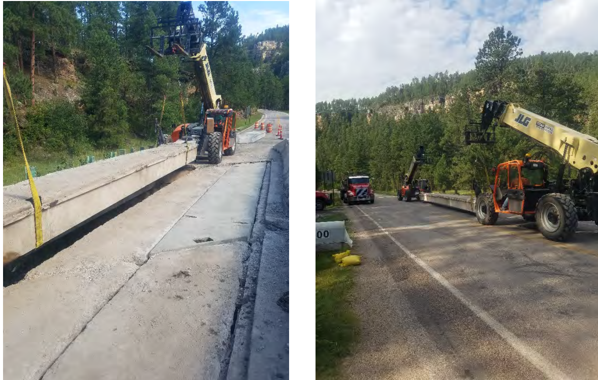
Figure 6.3 Extraction and Transportation of Salvaged Double-Tee Girders
