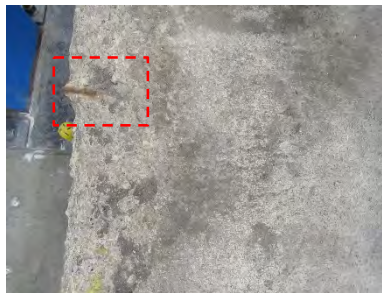
(w) Flange Exposure of Rebar (CS-2)
