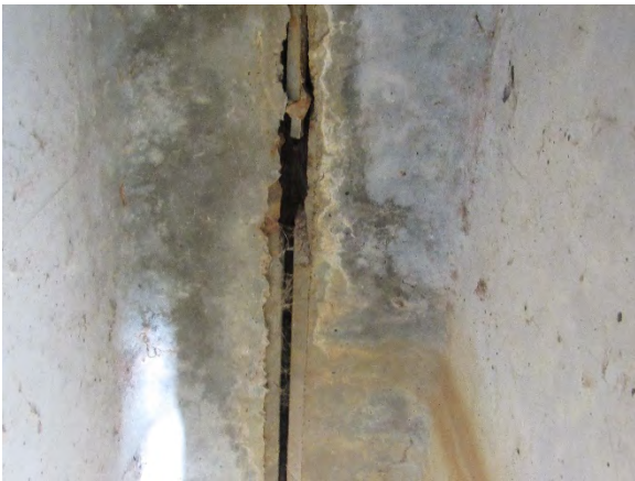
(c) Joint deterioration
