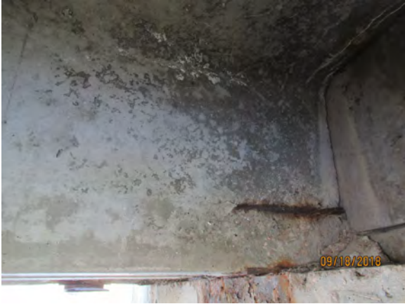
(f) Spall with Prestressing Strand Exposed – South End of East Stem of Deck Unit 6
