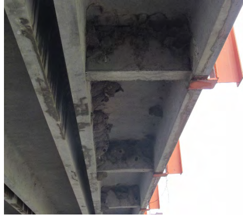
(b) Diaphragm at the exterior girder
