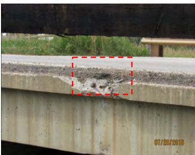
(v) Flange Exposure of Rebar (CS-1) & Flange Cover Deterioration (CS-4)
