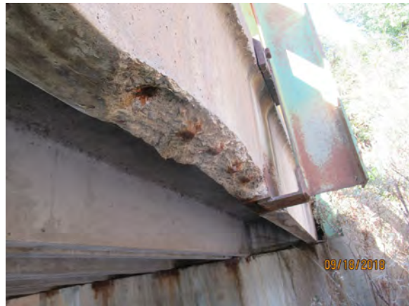
(i) Spall Near Rail Post 5 – Deck Unit 7
