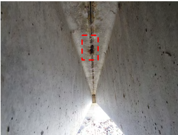
(c) Corrosion in the joint
