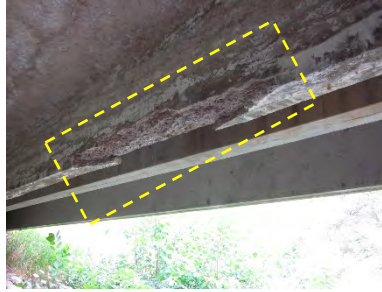
(b) Stem Cover Deterioration (CS-3)
