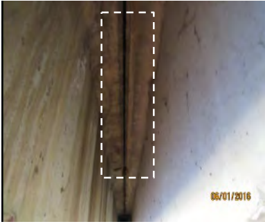
(m) Flange Girder to Girder Longitudinal Joint Deterioration (CS-2)
