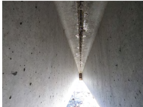
(f) Leakage from joint
