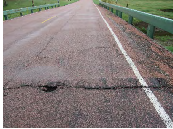
(b) Cracking on pavement over the bridge
