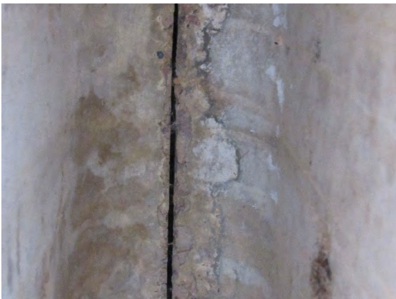
(e) Efflorescence at joint
