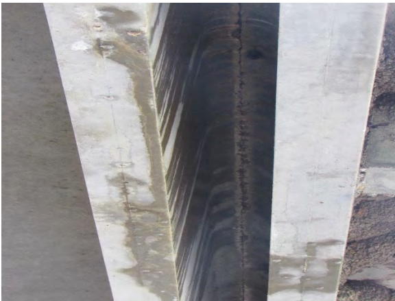
(c) Leakage from joint
