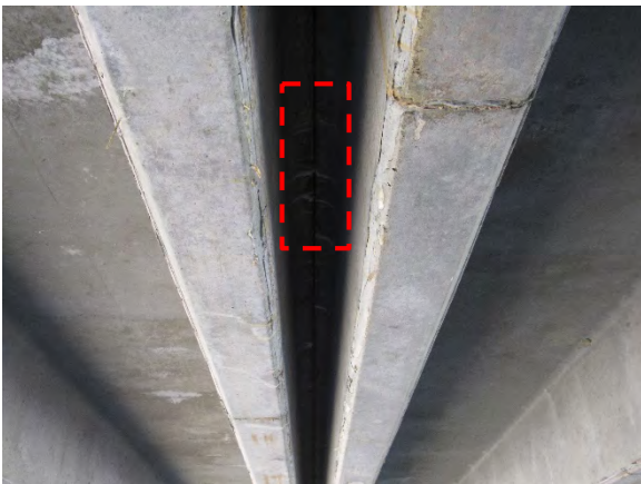
(e) Efflorescence at joint
