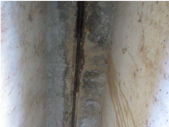
(e) Leakage from joint
