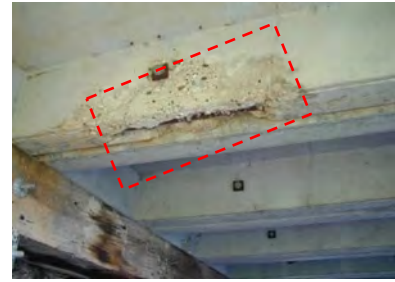
(c) Stem Cover Deterioration (CS-4)
