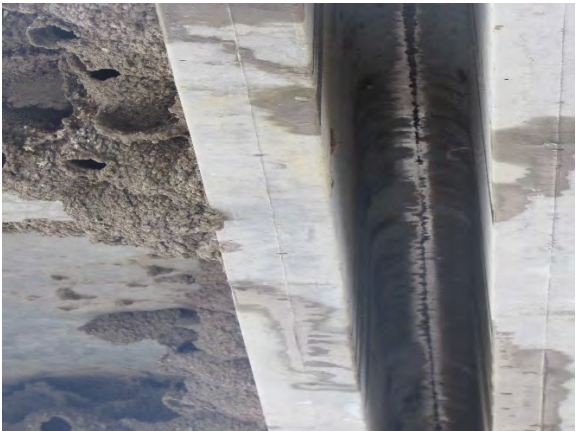
(e) Efflorescence in joint
