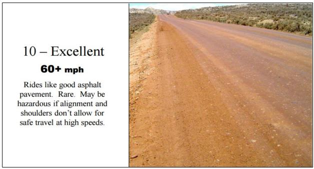
Figure 2.9 Gravel road with excellent conditions (Wyoming Technology Transfer Center, 2014)
