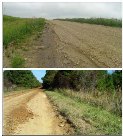
Figure 2.6 High Shoulders on road surface causing drainage issues (Federal Highway Administration, 2015)
