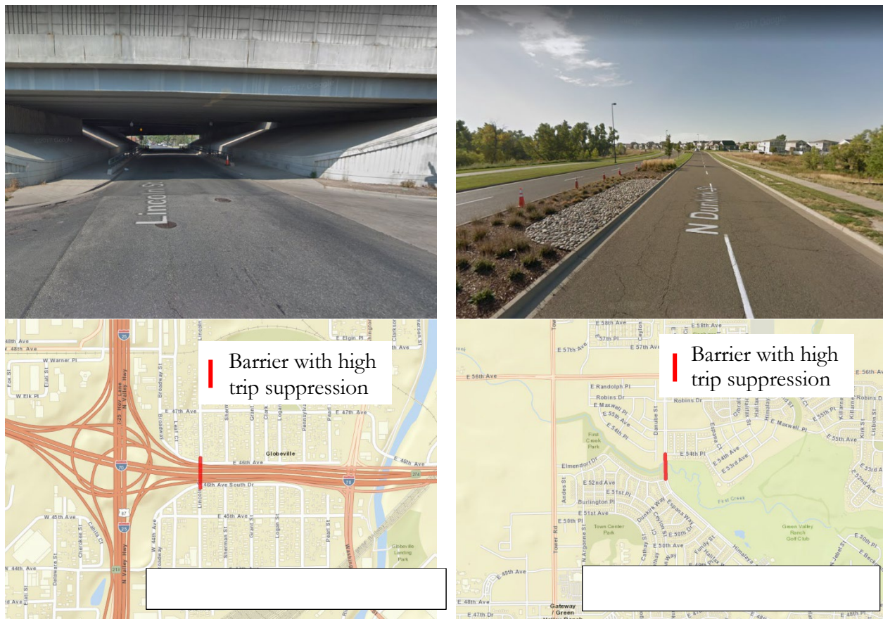
Figure 12.1 Examples of Barrier Connections with High Trip Suppression (Lincoln Street under I-70 on the left; Dunkirk Street over First Creek on the right)
