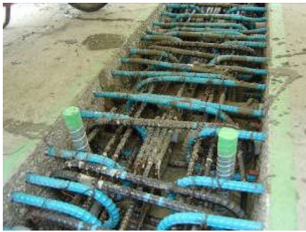
(a) Photograph of Longitudinal Joint
