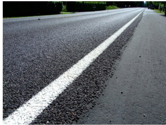
(b) Asphalt Chip Seal (after Gruen-Wald 2011)
