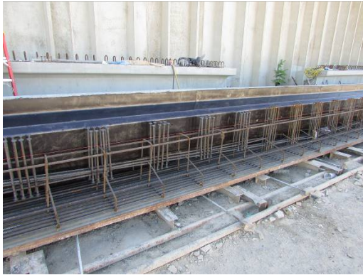
(a) Placement of Bars and Prestressing Strands
