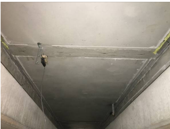
(a) Joint with Non-Shrink Grout – Deck Underneath
