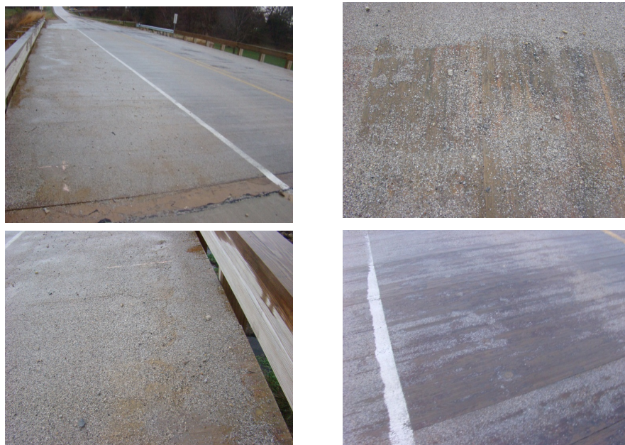
Figure 3.29 Epoxy with Embedded Grit Wearing Surface for Glulam Timber Bridge in Buchanan County, Iowa
