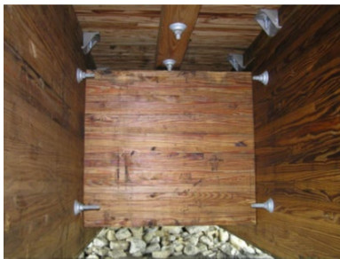
(a) Solid Glulam Diaphragm, (after Hosteng, 2013)
