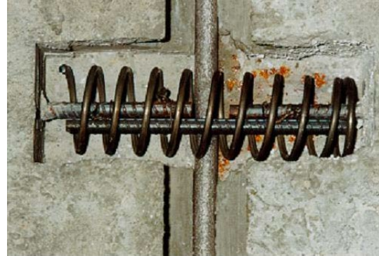
(b) Photograph of Block-out with Tied-in Lap Splice and Spiral Confinement (Badie et al., 1998)
