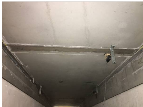
(b) Joint Latex Modified Concrete – Deck Underneath
