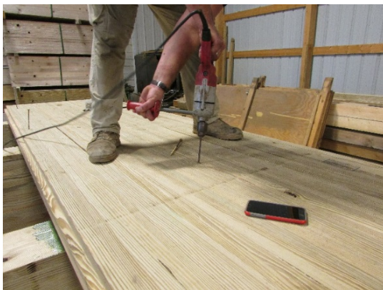
(c) Drilling GRK Screws
