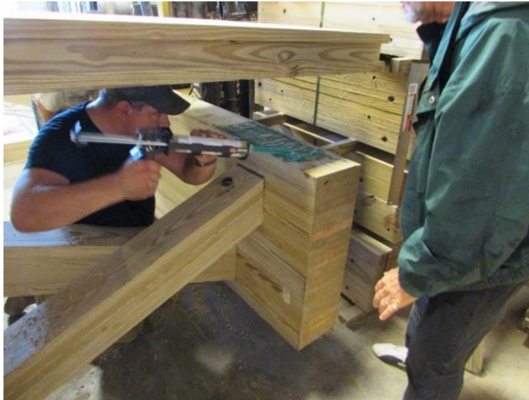
Figure 3.23 Epoxy Deck-to-Stringer Connection
