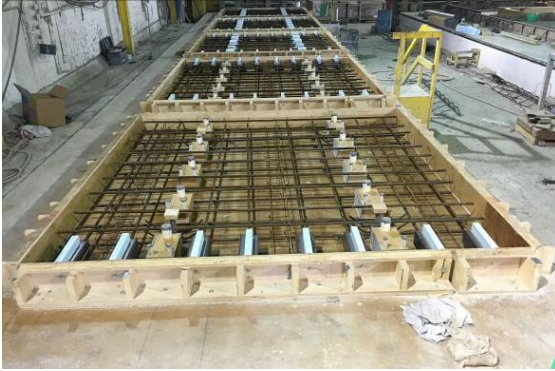
(a) Panel Formwork
