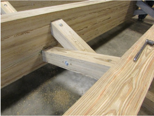
(a) Installation of Cross Braces
