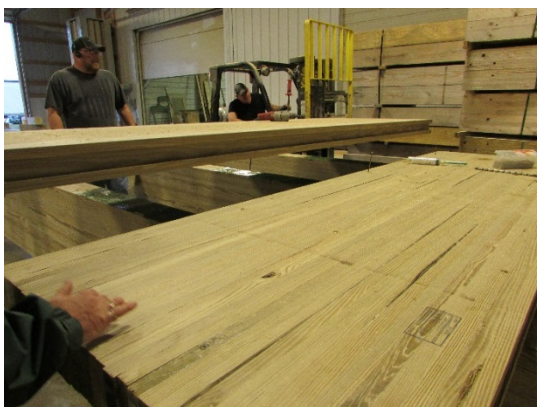
(e) Placement of Second Panel
