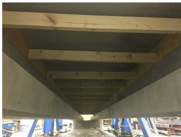
Figure 5.4 Grouted Haunch Region Formwork Installed between Girders
