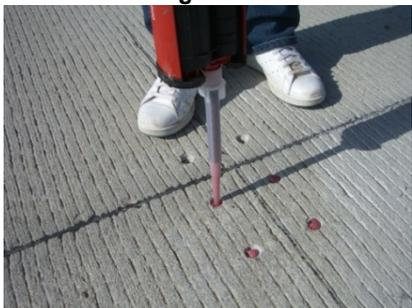
**Filling holes with epoxy adhesive**
