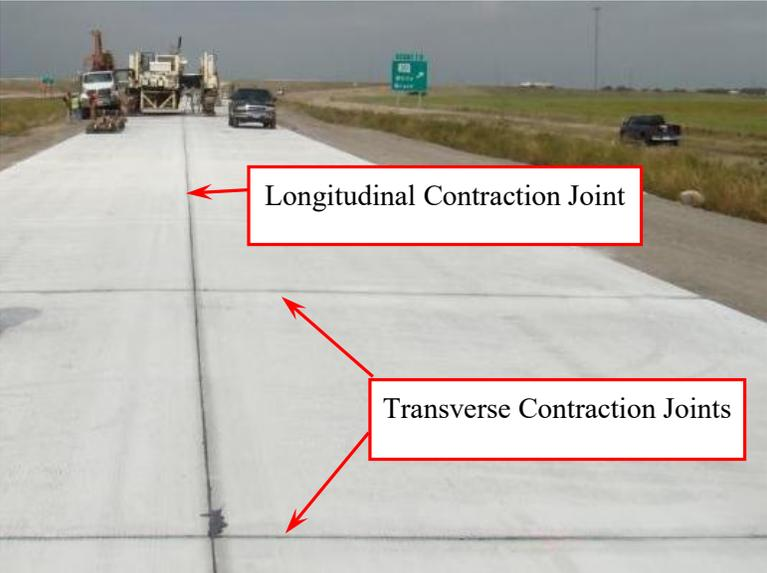
**Figure 1.1** JPC Pavement North of Brookings, SD
