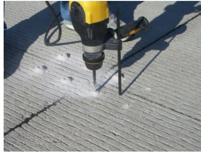
**Drilling 5/16-inch diameter holes**
