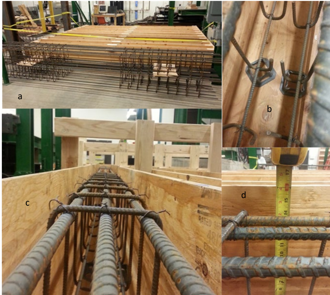
Figure 2.12 a) Rebar cages, b) 40mm plastic rebar chairs, c) position of rebar cage in form, d) depth of tensile reinforcement once supported on 40mm rebar chairs
