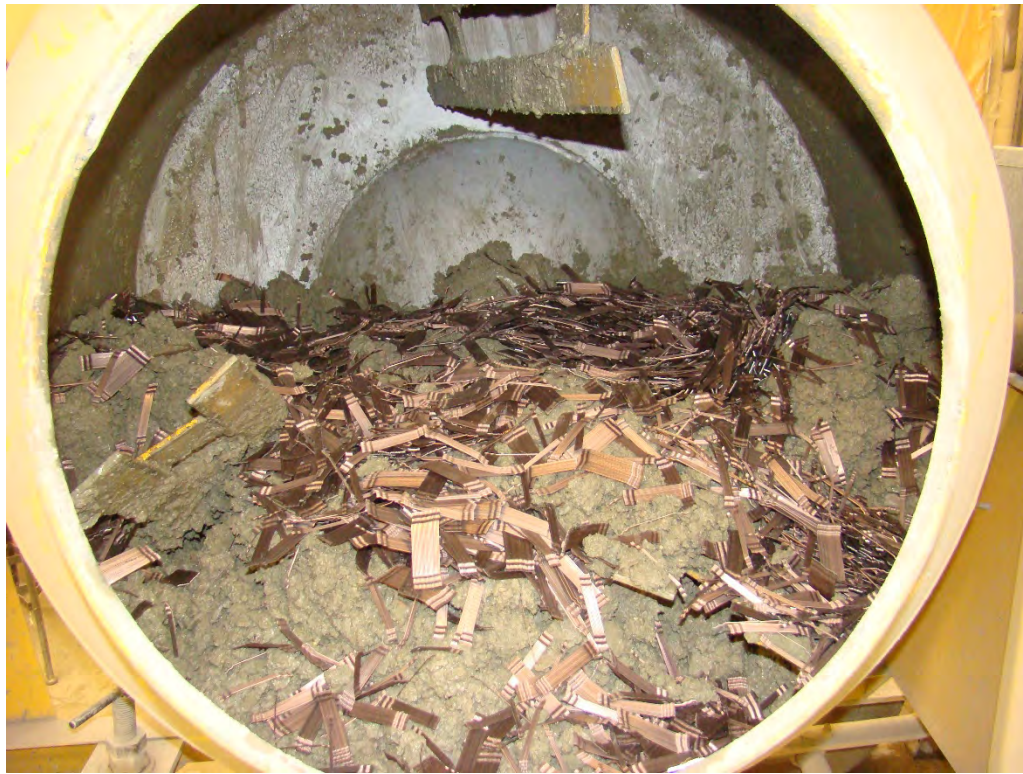
Figure 5.8 Distribution of fibers on the surface of the resting concrete, prior to the final five minutes of mixing
