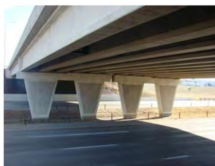
**(d)** Flared-Column Bent**Figure 3.19** Typical Bridge Bents in Collision Risk Quadrants 4-4, 3-4, and 4-3
