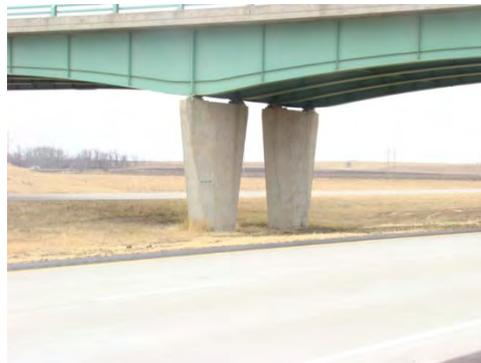
**Figure 3.10** Flared Columns with No Bent Cap
