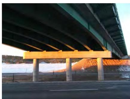
**(c)** Three-Circular Column Bent
