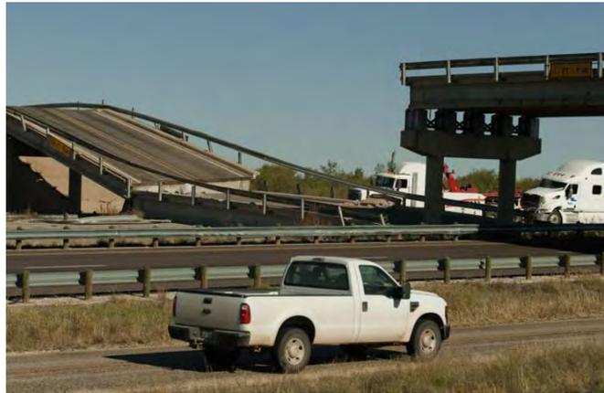
**Figure 3.3** I-80 Bridge Collapse near Big Springs, TX (Midland Reporter Telegram, 2013)
