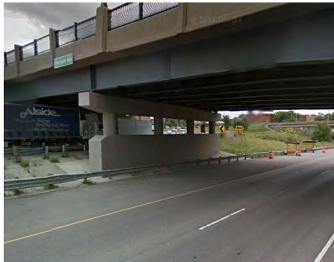
**Figure 3.22** Crash Strut Retrofit (Courtesy MnDOT)
