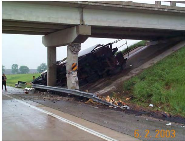
**Figure 3.4** I-90 Bridge Collision near Worthington, MN
