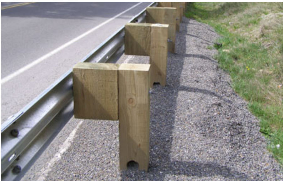
Figure 2.3 Semi-Rigid Barrier System: Strong Post W-Beam (Source: safety.fhwa.dot.gov )
