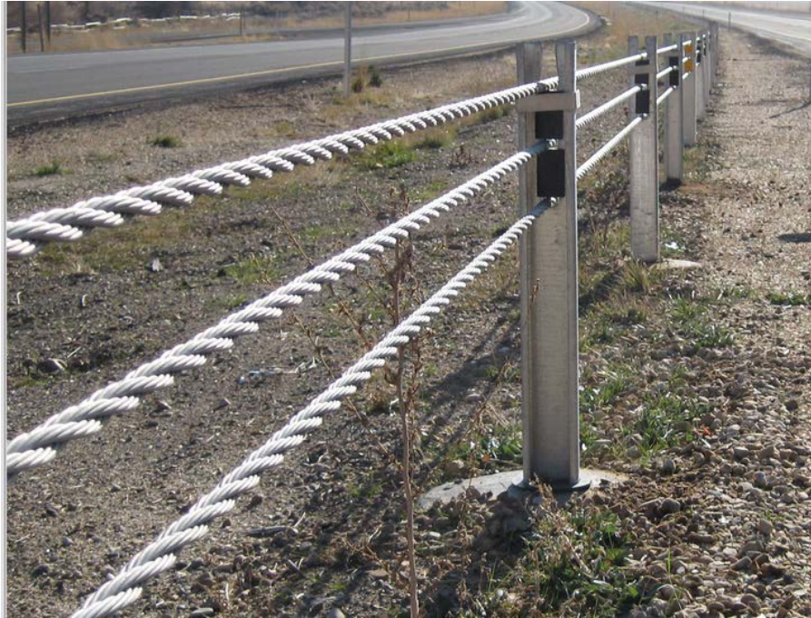
Figure 2.4 Flexible Barrier System: Three-Strand Cable (Source: blog.udot.utah.gov )
