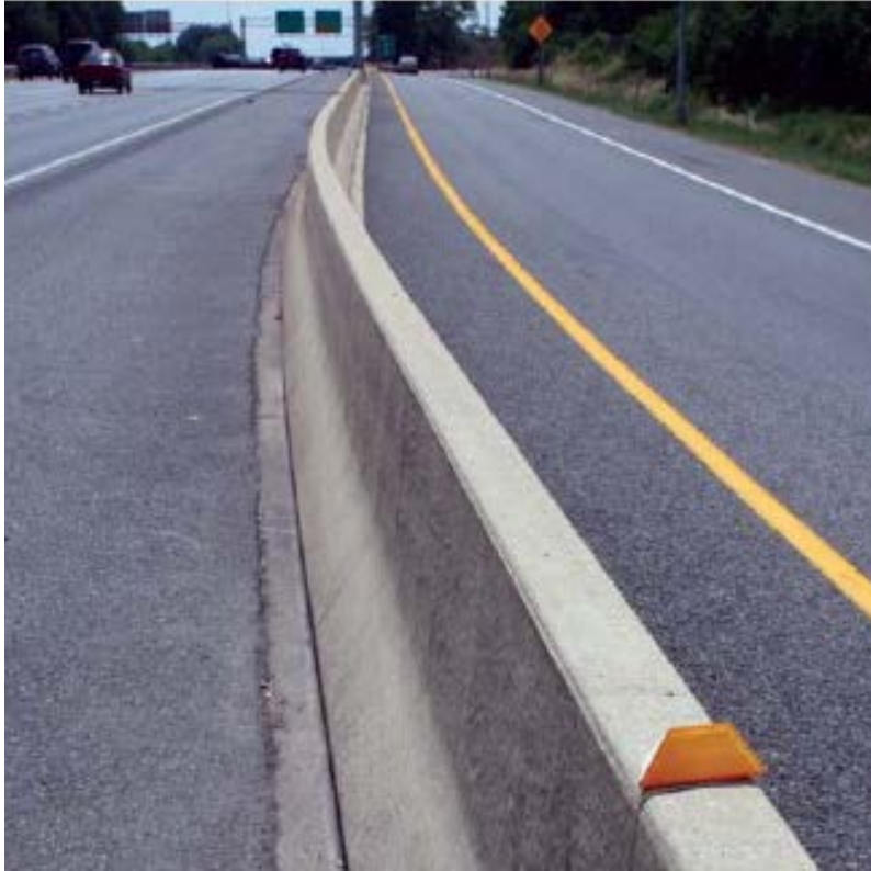
Figure 2.4 Rigid Barrier System: Concrete (Source: safety.fhwa.dot.gov )
