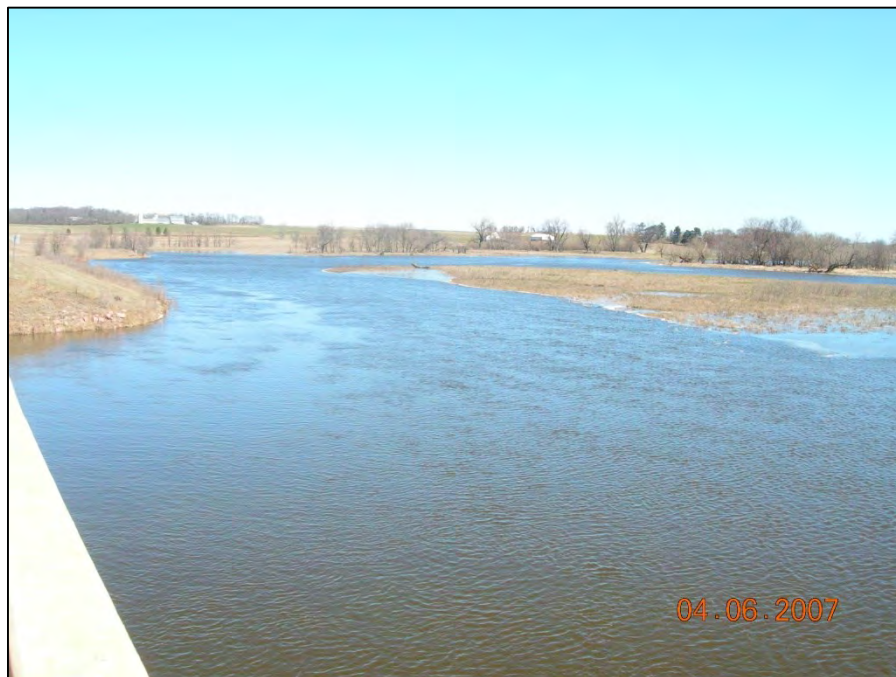
Figure 4.3 From SD 13 Bridge facing upstream toward the right bank. Note the 90° bend in the channel in front of the bridge
