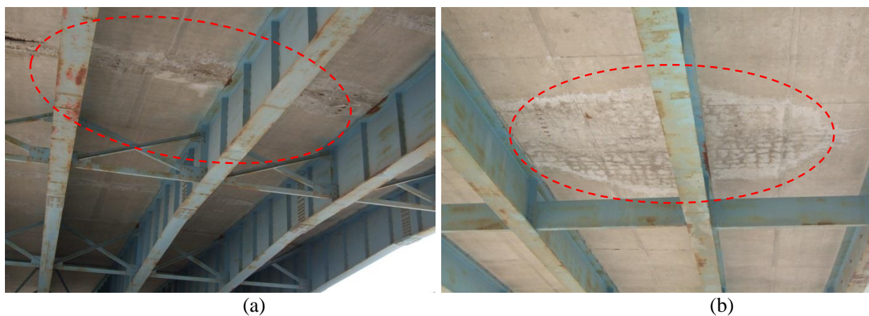
Figure I.3 Deteriorated bridge decks in I-29, North Dakota: (a) corrosion and concrete-spalling; (b) repaired deck
