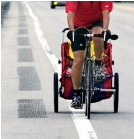
Figure 2.2 Intermittent Rumble Strips on 3 ft. Shoulders
