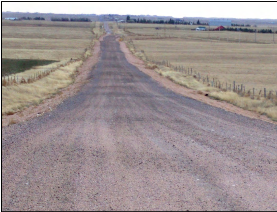
Figure 4.11 Segregation bands attributed to inadequate spreading of the windrows placed by the bottom-discharge haul trucks on Laramie County's Pry Road in November 2008, six months after initial application.
