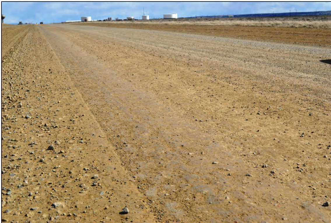
Figure 4.32 Road surface made of limestone crushed base treated with magnesium chloride on Sweetwater County's Crooks Gap Road.
