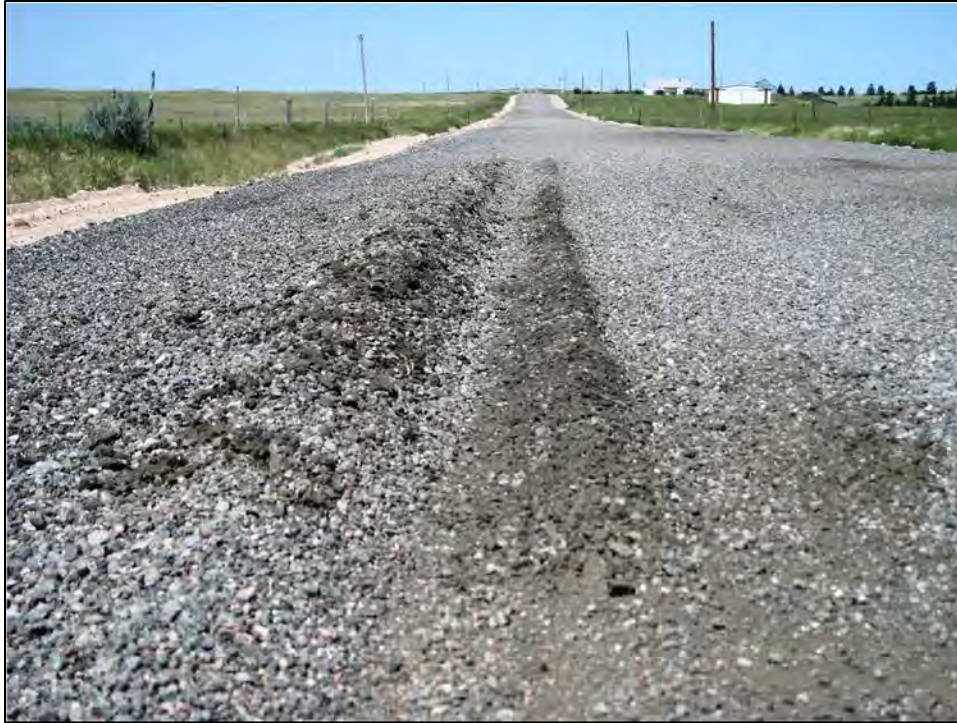
Figure 4.12 Nearly 100% RAP resulting in excessive loose aggregate on Laramie County's Atlas Road in June 2008, about two months after initial application.
