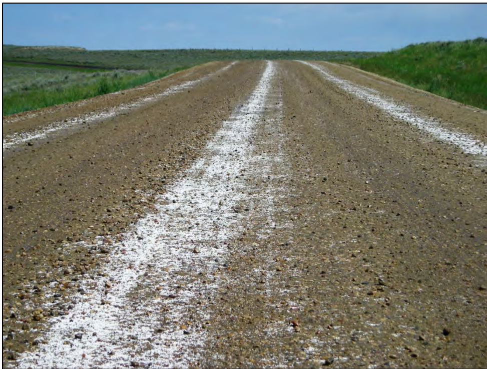
Figure 3.28 Calcium chloride flakes partially worked into the aggregate surface by traffic on Johnson County's Schoonover Road, June 2008.
