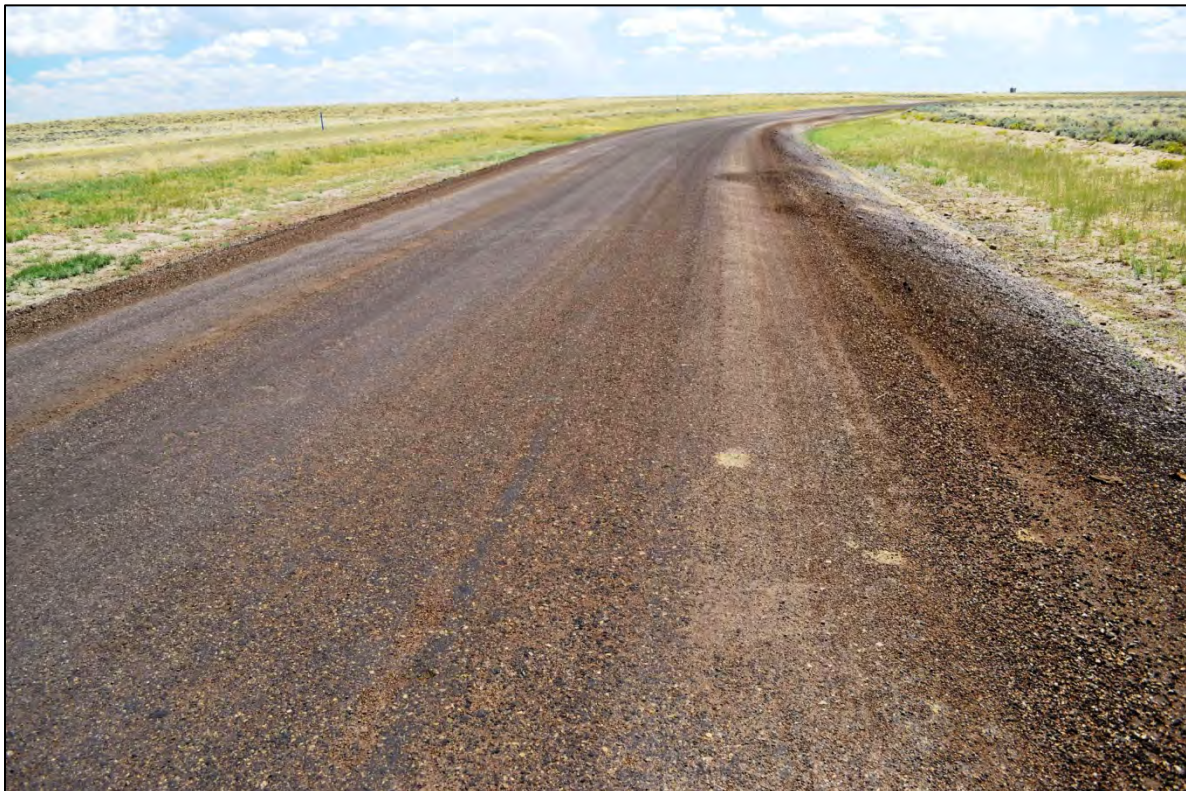
Figure 4.48 Road surface made from RAP blended with existing aggregate and treated with magnesium chloride on segment of Sweetwater County's Crooks Gap Road in August 2011, three weeks after application of dust suppressant.
