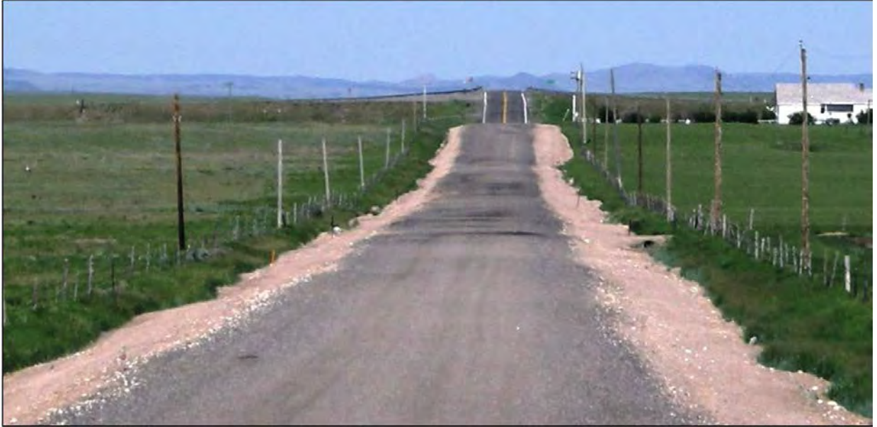
Figure 4.10 Segregation of RAP on Laramie County's Atlas Road in June 2008, two months after initial RAP application.
