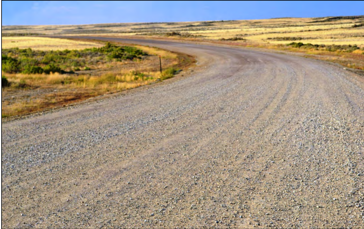
Figure 4.38 Broken up crust of limestone crushed base, foreground, and still intact crust, background, both treated with lignin and magnesium chloride on uphill, curved segment D of Sweetwater County’s Crooks Gap Road in September 2011, eight weeks after application of dust suppressant.
