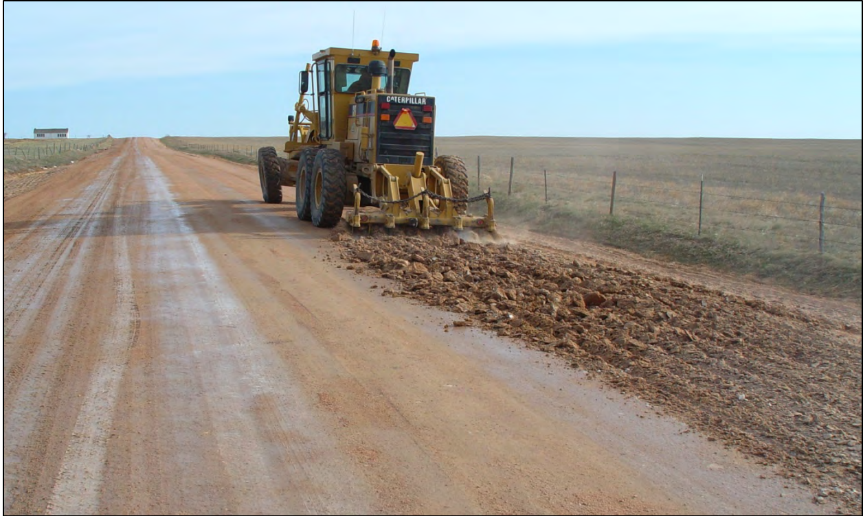
Figure 3.16 Scarifying Laramie County's Atlas Road prior to placement and blending of RAP.
