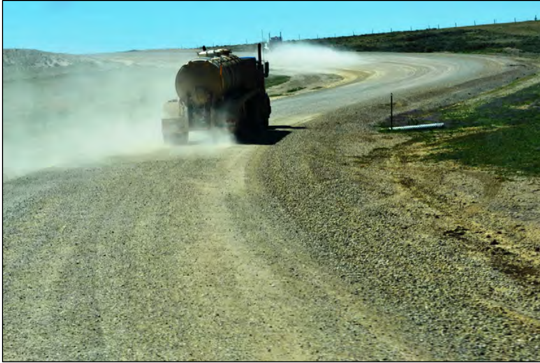
Figure 4.34 Dust from limestone crushed base before dust suppressant application on uphill, curved segment D of Sweetwater County's Crooks Gap Road in June 2011.
