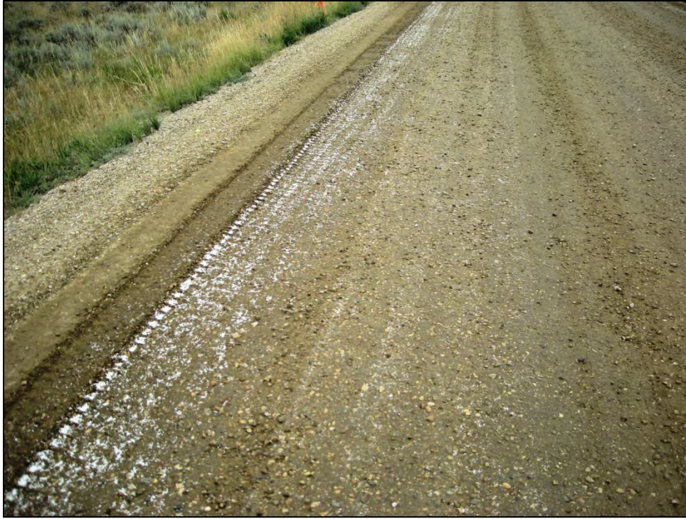
Figure 3.29 Calcium chloride flakes mostly worked into the aggregate surface by traffic on Johnson County's Schoonover Road, June 2008.
