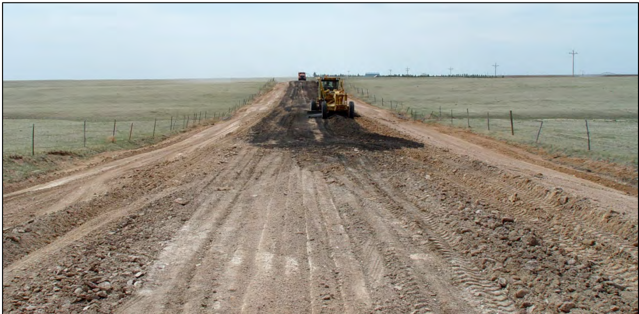
Figure 3.19 Blending and shaping RAP and existing, scarified aggregate on Laramie County's Atlas Road.
