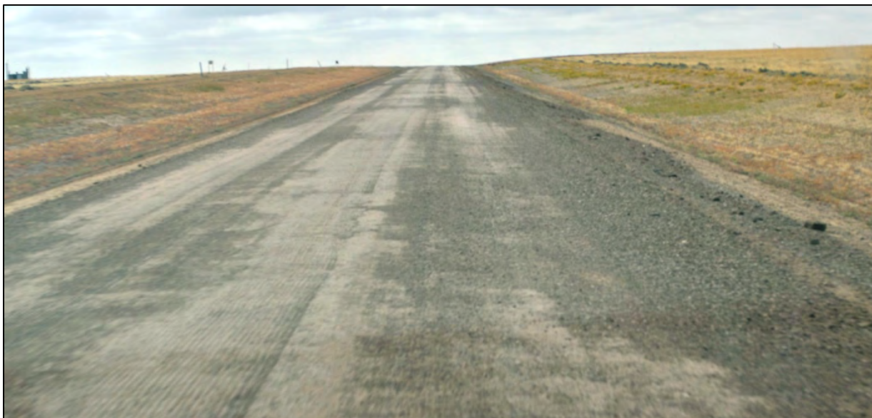
Figure 4.52 Road surface made with RAP blended with existing aggregate on segment P of Sweetwater County's Crooks Gap Road in September 2011.
