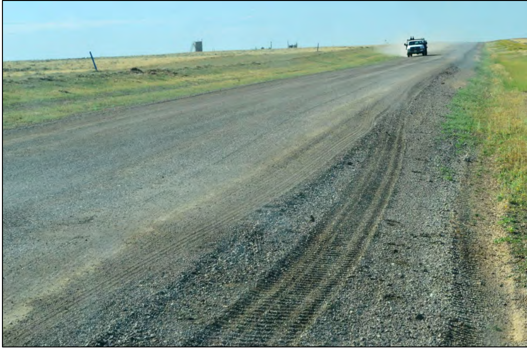
Figure 4.49 Road surface made from RAP blended with existing aggregate on segment P of Sweetwater County's Crooks Gap Road in August 2011.
