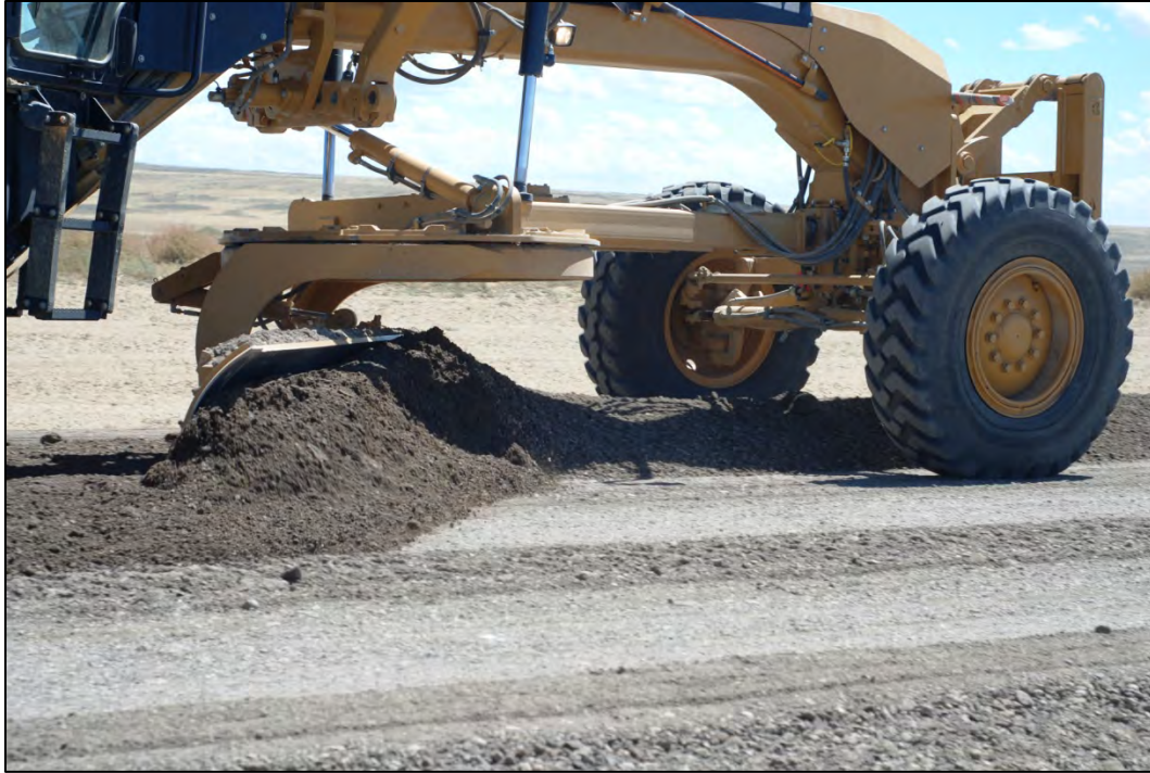
Figure 3.32 Blending and shaping the existing aggregate and CTB blend on Sweetwater County's Crooks Gap Road, August 2010.
