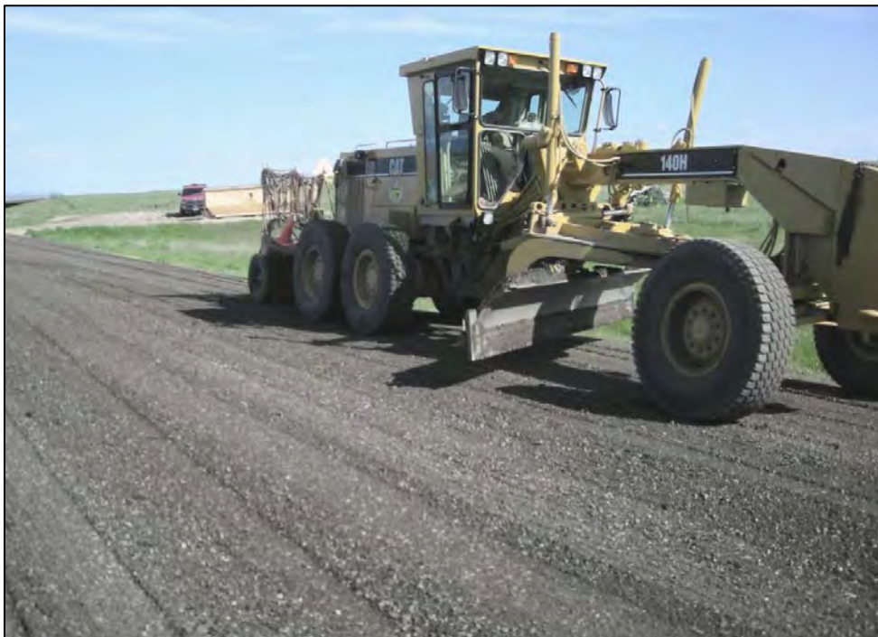
Figure 3.24 Compacting RAP and aggregate blend on Johnson County's Schoonover Road with pneumatic tire compactors mounted on the motor grader's ripper hydraulics, June 2008.
