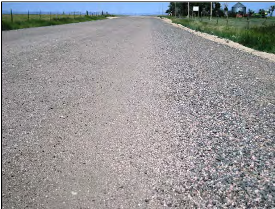
Figure 4.13 Well compacted, tight surface due to good blending on Laramie County's Atlas Road in June 2008, about two months after initial application.
