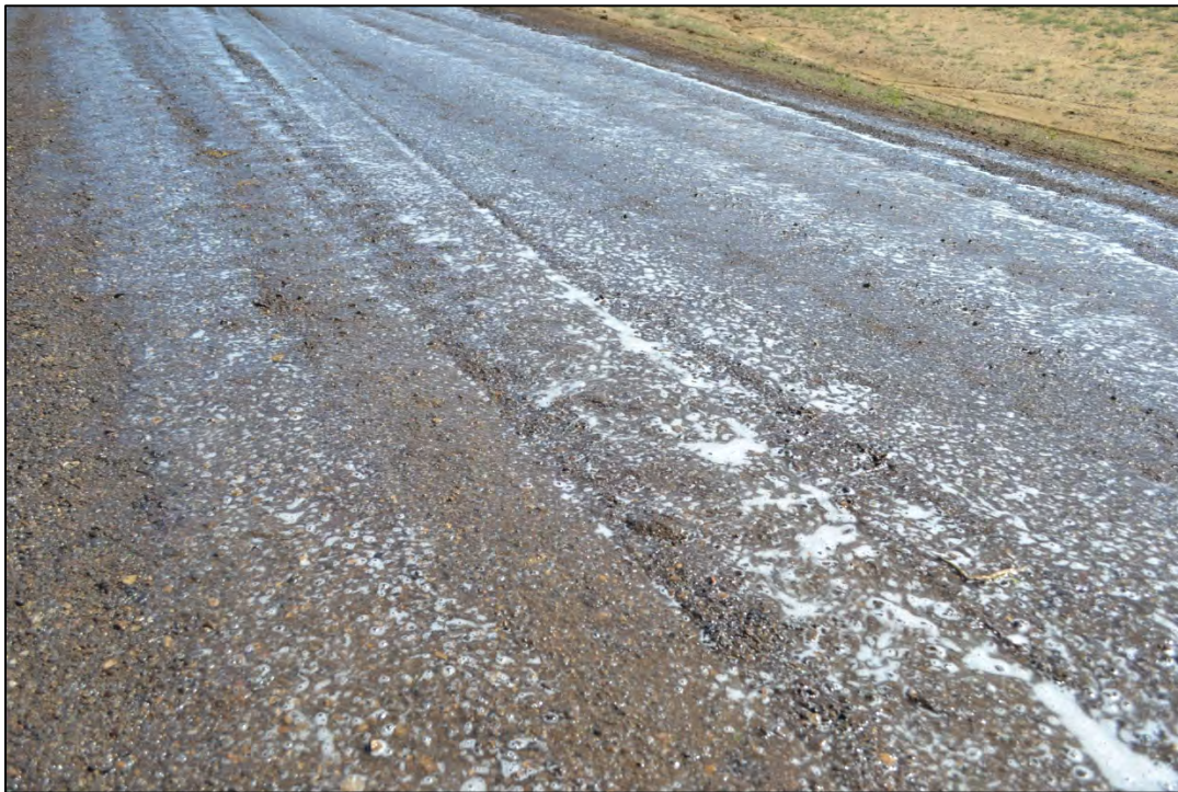
Figure 3.38 Recently applied magnesium chloride on the RAP and aggregate blend on Sweetwater County's Crooks Gap Road, July 2011.
