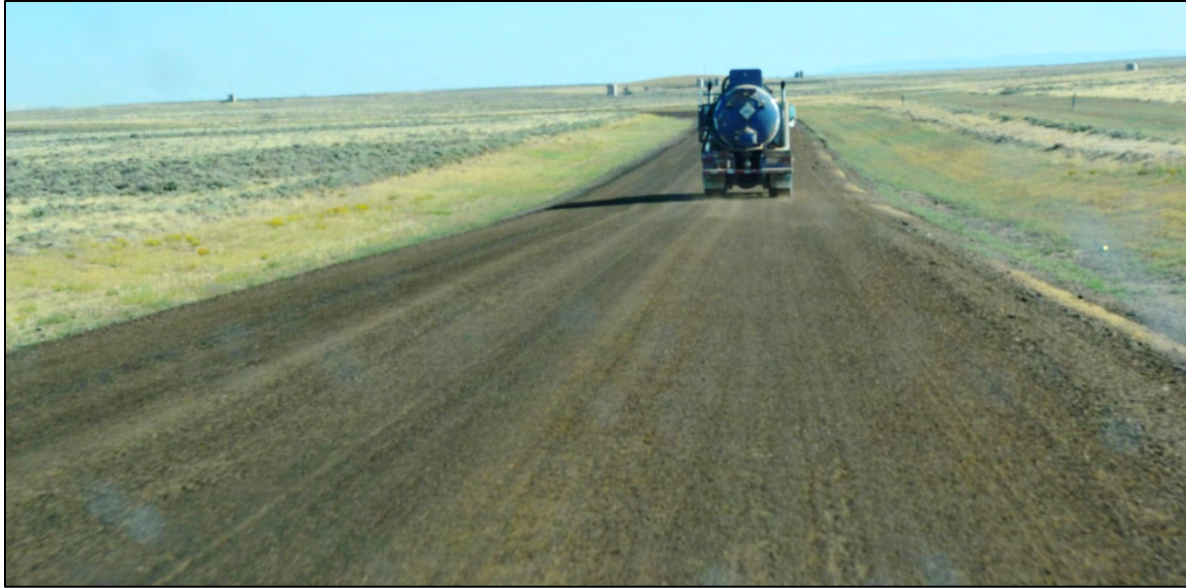
Figure 4.47 Road surface made from RAP blended with existing aggregate treated with magnesium chloride and polymer on segment M of Sweetwater County's Crooks Gap Road in August 2011, three weeks after application of dust suppressant.
