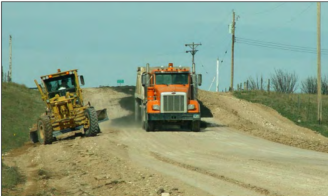
Figure 3.17 Placement of RAP windrow on Laramie County's Atlas Road with bottom-discharge haul trucks.
