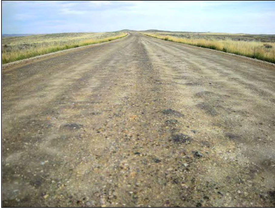
Figure 4.24 Road surface on Johnson County's Schoonover Road, segment S1 with RAP and calcium chloride in October 2008, four months after RAP placement and three months after calcium chloride application.
