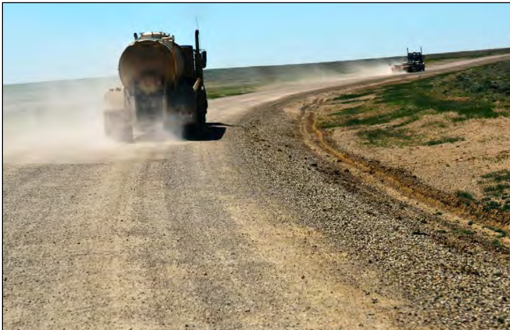
Figure 4.35 Dust from limestone crushed base before dust suppressant application on level, curved segment C on Sweetwater County's Crooks Gap Road in June 2011.
