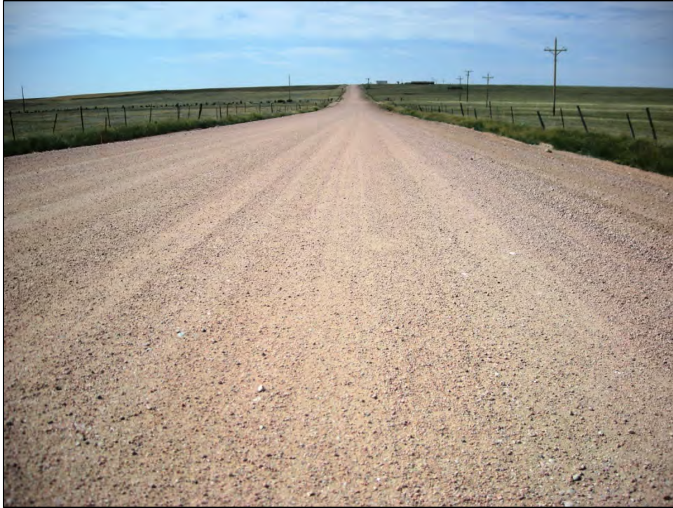
Figure 4.17 Aggregate only forming a good driving surface on Laramie County's Pry Road in July 2008, two months after shaping.
