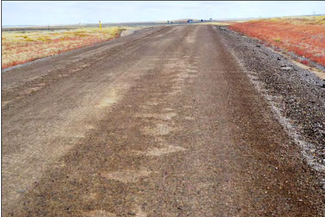
Figure 4.51 Road surface made with RAP blended with existing aggregate and treated with magnesium chloride and polymer on segment L of Sweetwater County's Crooks Gap Road in September 2011, eight weeks after application of dust suppressant.
