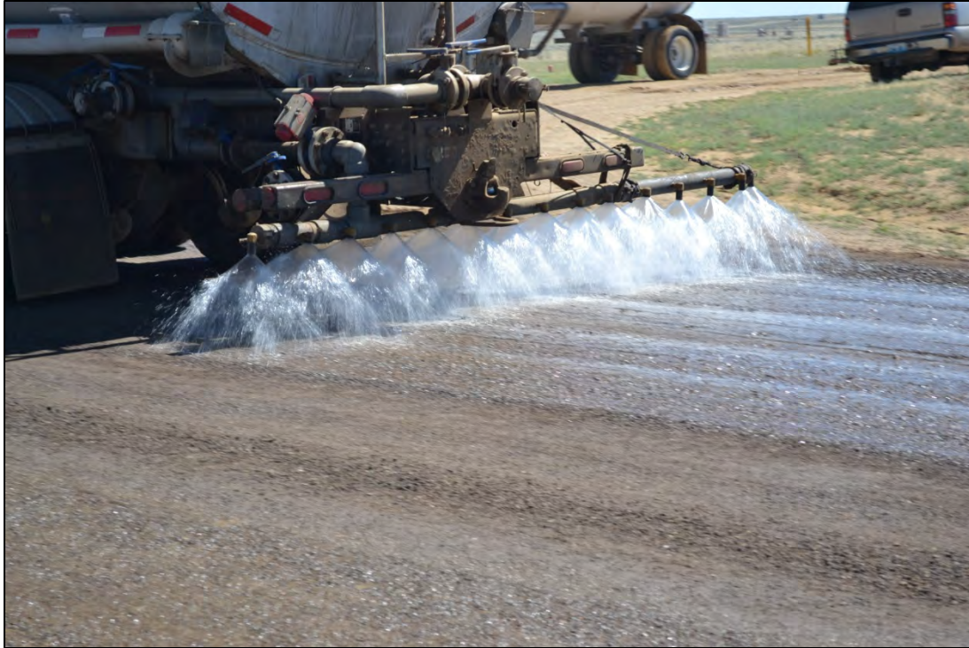
Figure 3.37 Applying dust suppressant brine to aggregate and RAP blend on Sweetwater County's Crooks Gap Road, July 2011.
