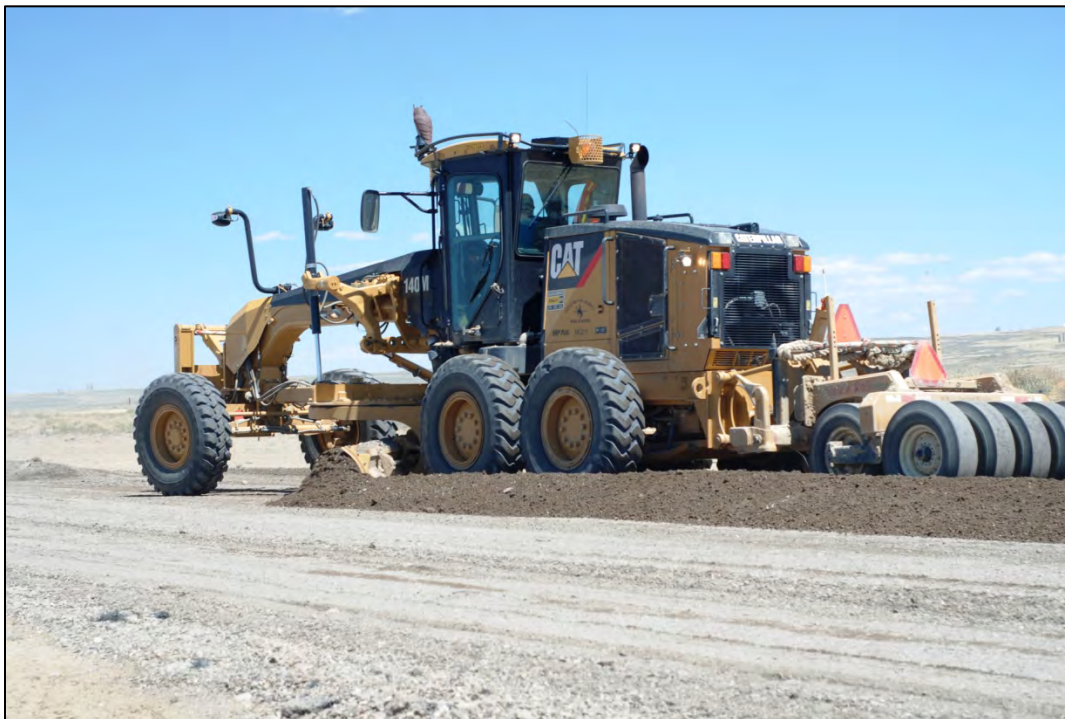
Figure 3.33 Final shaping and compaction of CTB and aggregate blend using a motor grader with pneumatic tire compactors mounted to its ripper hydraulics on Sweetwater County's Crooks Gap Road, August 2010.
