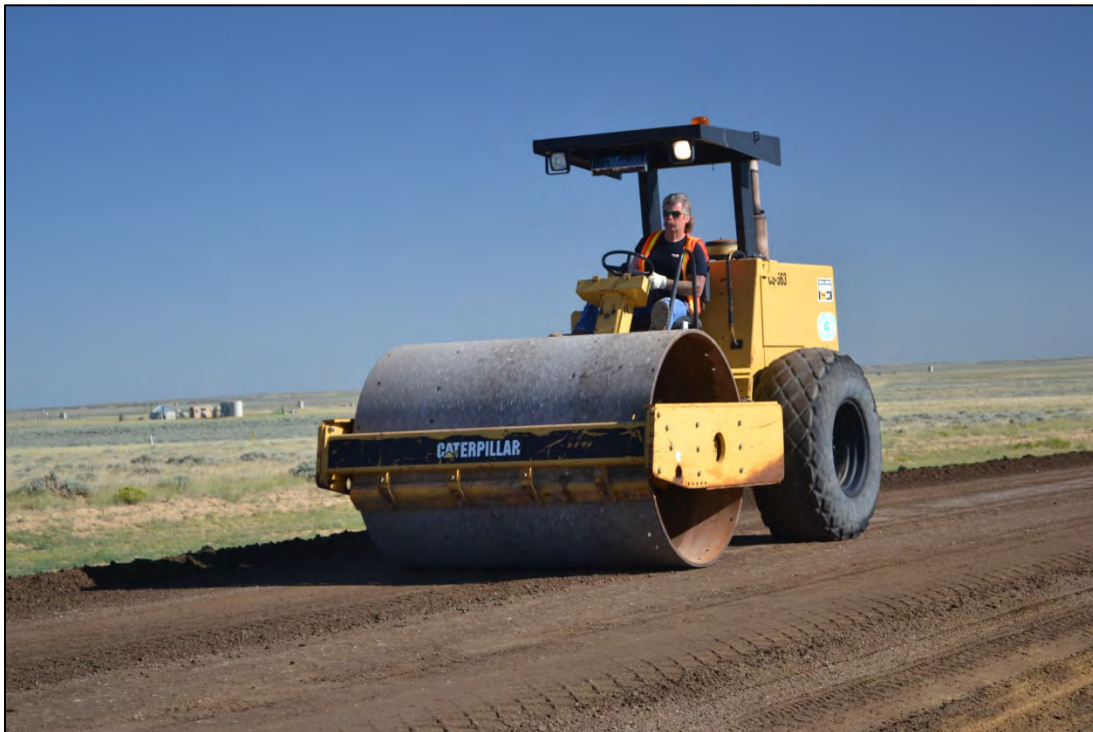
Figure 3.40 Compaction of the magnesium chloride-treated RAP and aggregate blend on Sweetwater County's Crooks Gap Road, July 2011.
