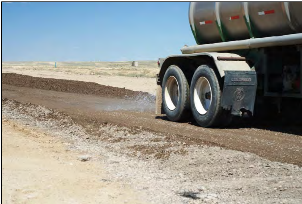
Figure 3.31 Applying water to the CTB and aggregate blend prior to final shaping and compaction on Sweetwater County's Crooks Gap Road, August 2010.
