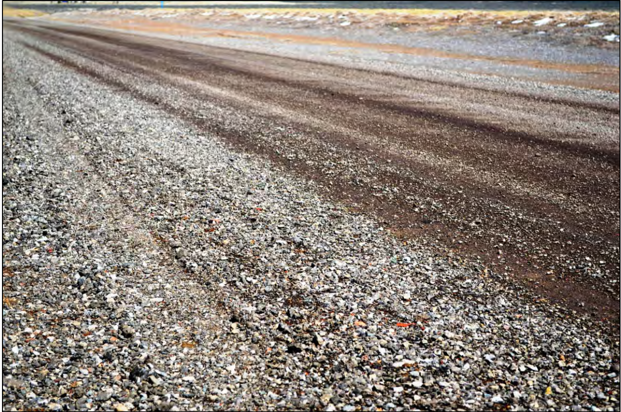
Figure 4.46 Road surface made from RAP blended with existing aggregate on segment Q of Sweetwater County’s Crooks Gap Road in April 2011 without dust suppression agents.
