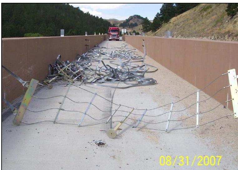
Figure 4.5 The crumbled wire gates following a successful ramp event.
