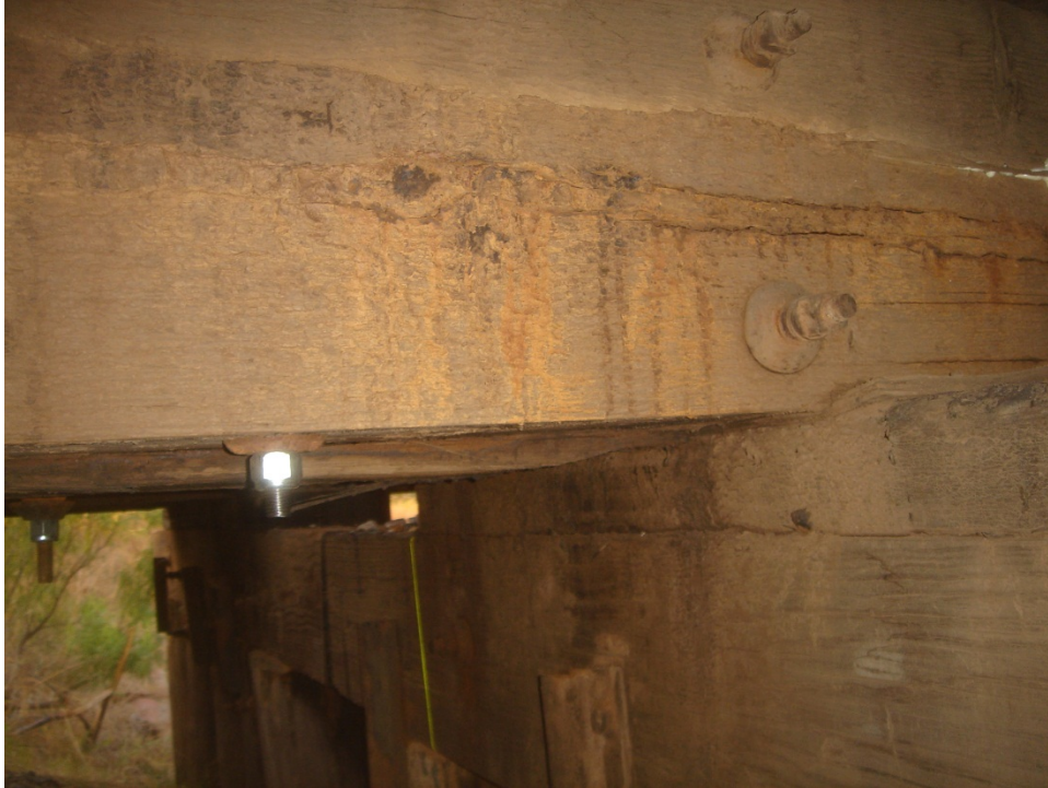
Figure C.25 View showing compressed Stringer 3, Span 1
