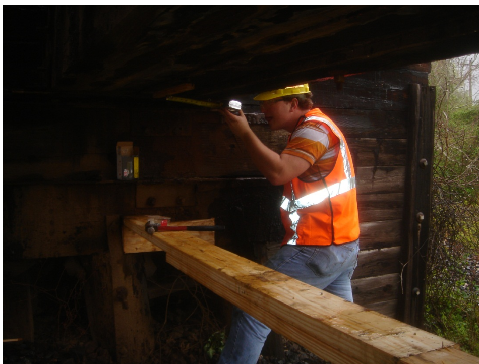
Figure B.4 Alternate base for String Potentiometers (Glidden Sub 69.11)
