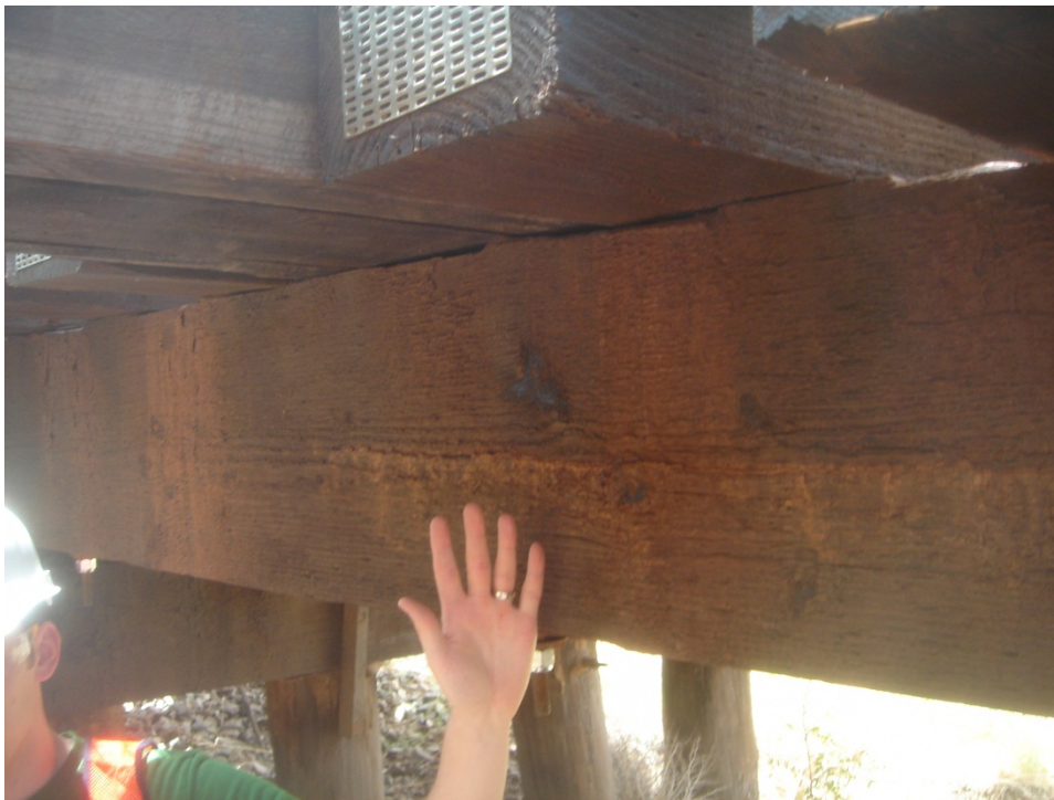
Figure C.10 Horizontal Shear Crack in Stringer 1, Span 2. Coded 4A
