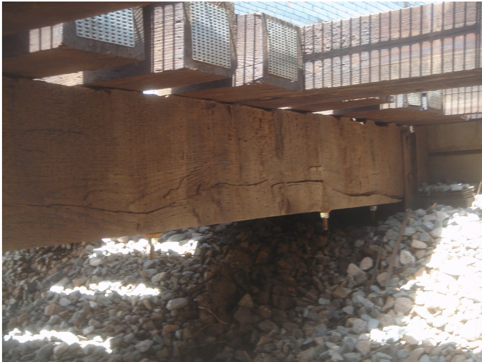
Figure C.4 Span 1, Stringer 1, badly cracked due to large knots and split near the abutment.
