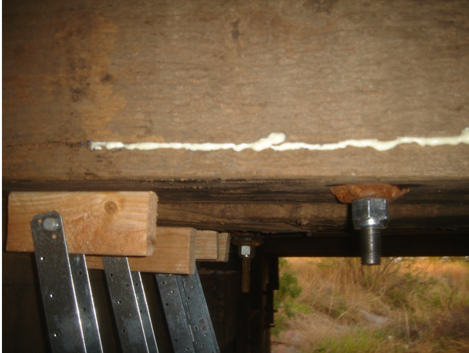
Figure C.37 Spray foam used to fill cracks
