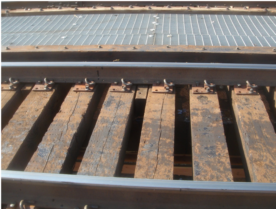
Figure C.44 Top view of spikes inserted in beams.
