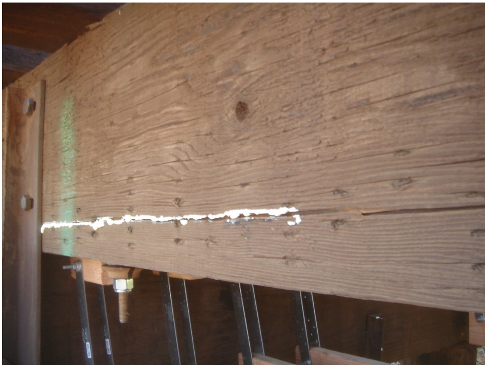
Figure C.38 Spray foam used to fill cracks
