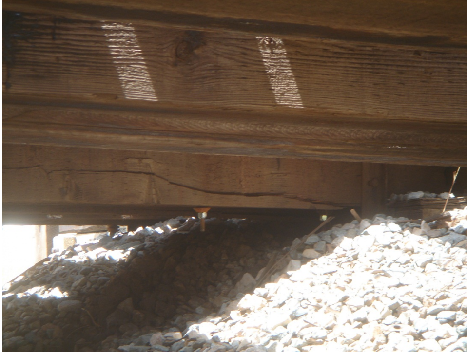
Figure C.5 Span 1, Stringer 1, badly cracked due to large knots and split near the abutment.
