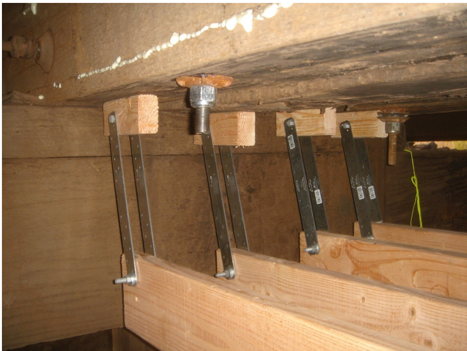
Figure C.26 View of showing compressed Stringer 3, Span 2
