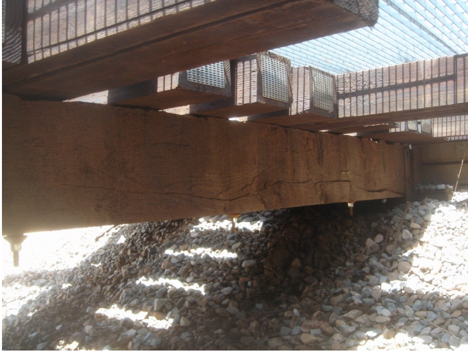
Figure C.3 Span 1, Stringer 1, badly cracked due to large knots and split near abutment.
