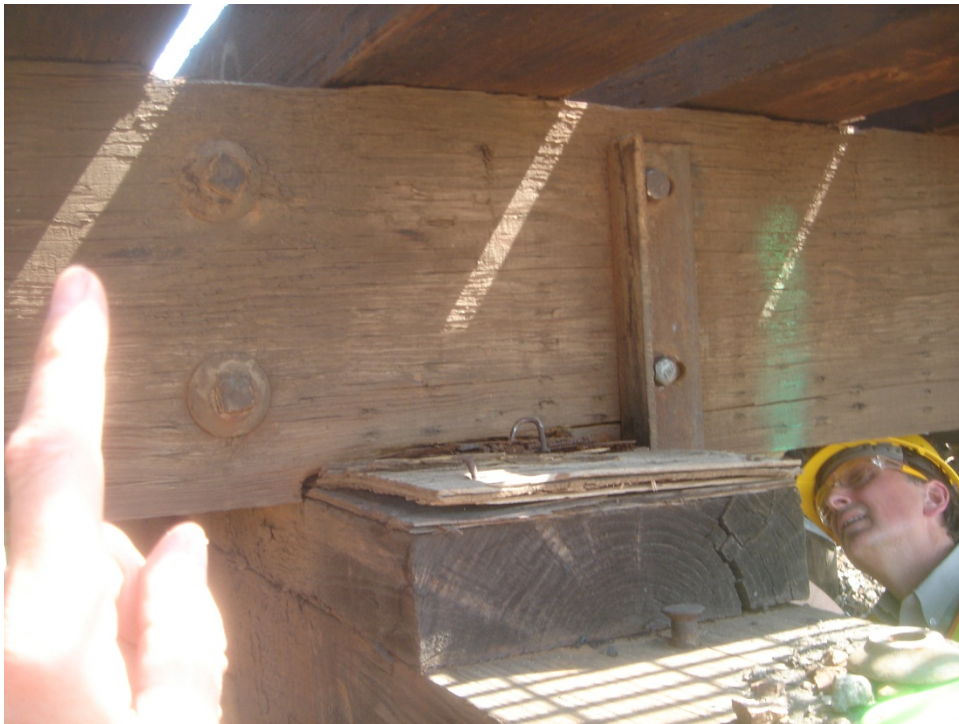
Figure C.32 Stringer 8 – Close up of damage over pier
