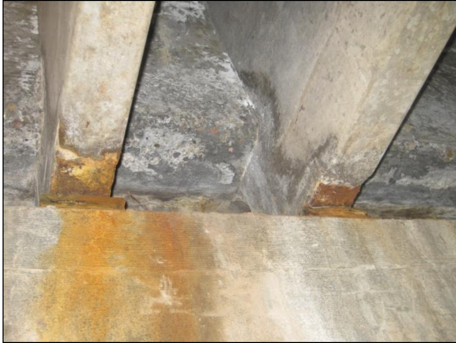
Figure E.25 Bridge 8 - Rust at supports
