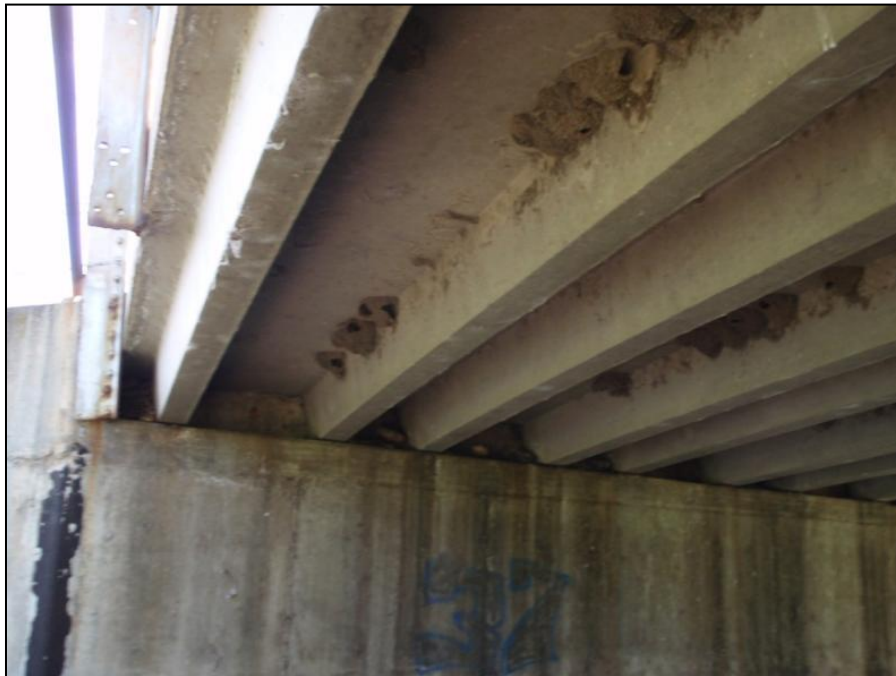
Figure E.39 Bridge 12 Double T-girders
