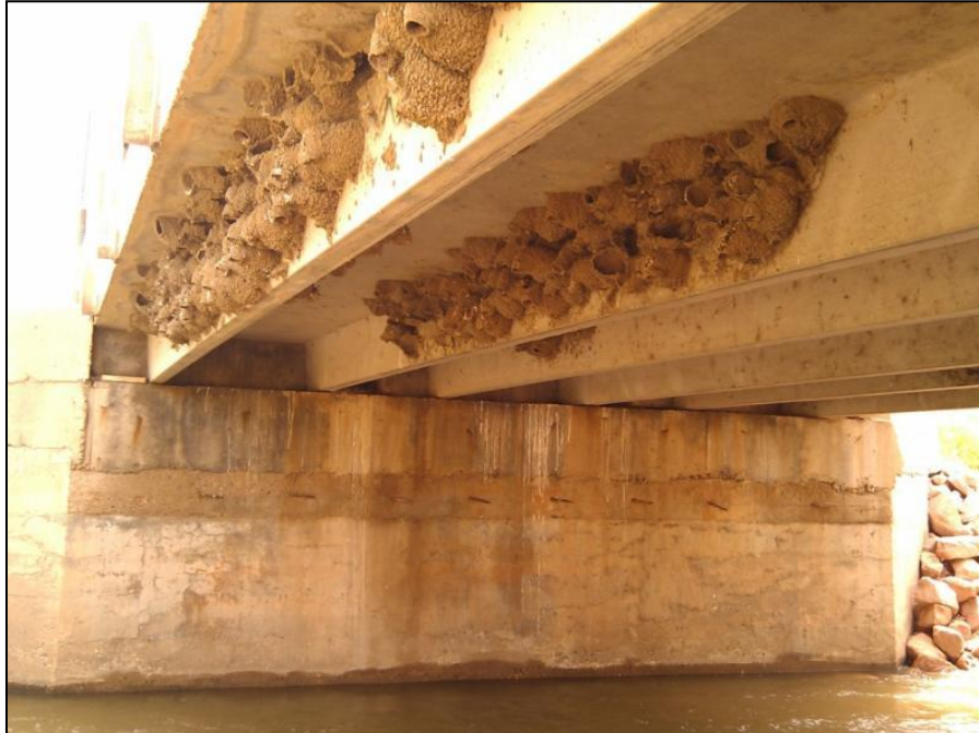
Figure E.45 Bridge 14 Double T-girders
