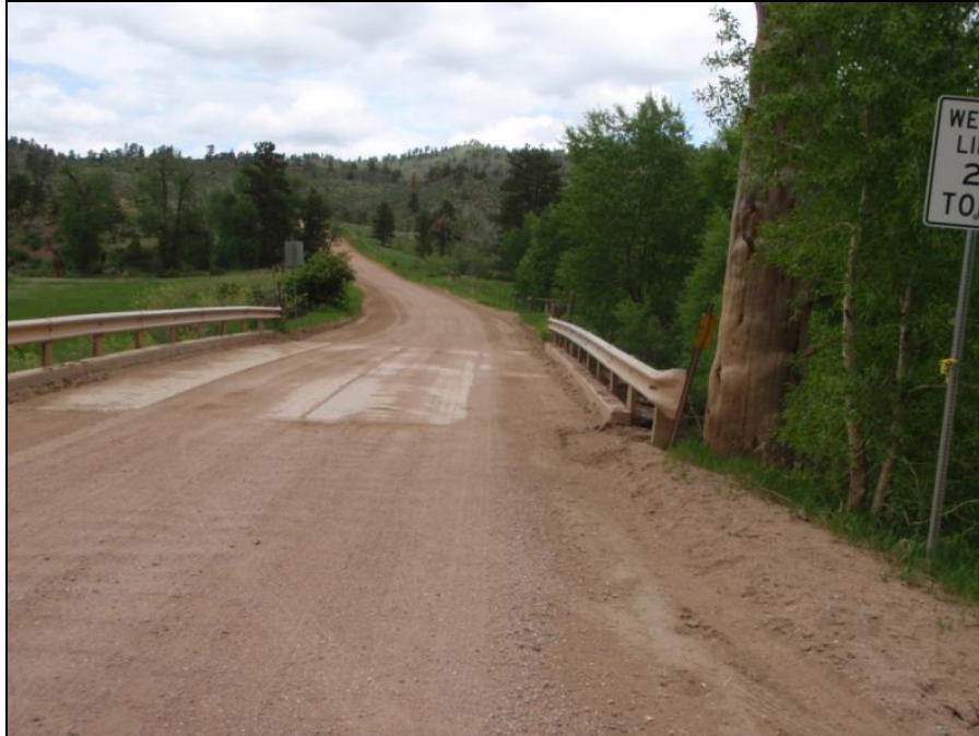
Figure E.56 Bridge 16 - Exposed Girder Flanges
