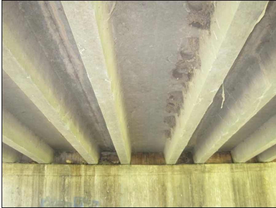
Figure E.42 Bridge 12 Double T-girders
