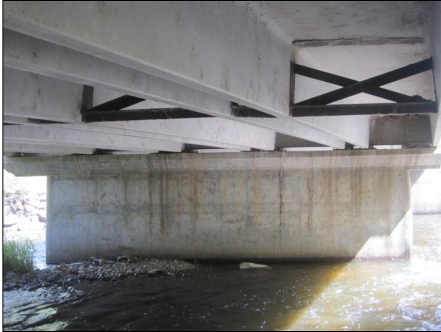
Figure E.34 Bridge 10 Double T- Girders
