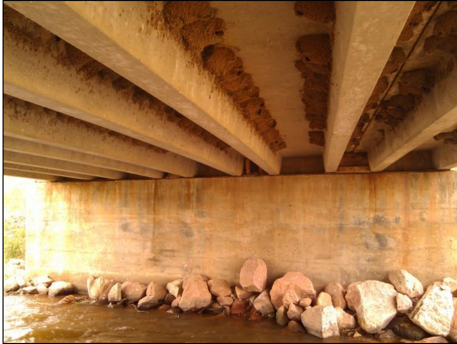
FigureE.5 Bridge 2 - Double T-beams
