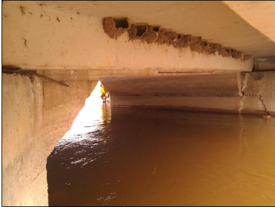
FigureE.52 Bridge 15 Widened with Double T-Girder
