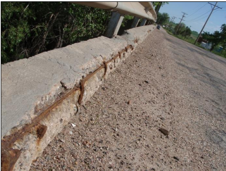
Figure E.2 Exposed Rebar on Bridge 1
