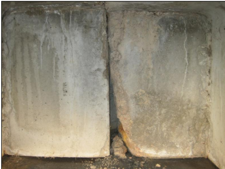
Figure E.16 Spalling of concrete on Bridge 6
