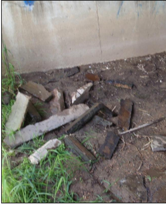
Figure 3.1 Concrete pieces from streambed underneath Bridge 12.
