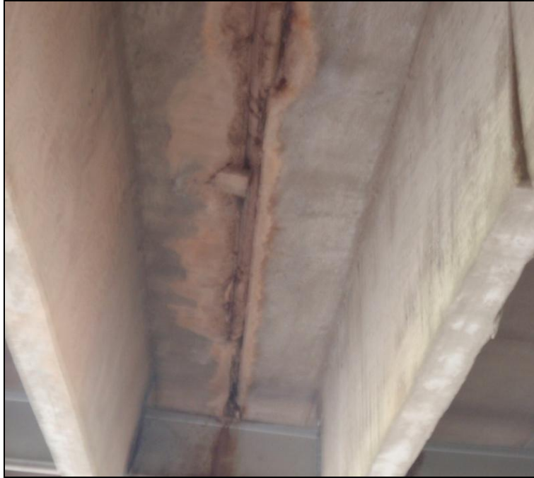
Figure E.58 Bridge 16 - Cracking at girder joint
